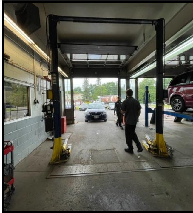
Photograph 9: Interior view of the garage showing the oil-water separator channel.
