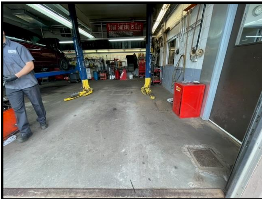
Photograph 8: Interior view of the subject building (service garage).
