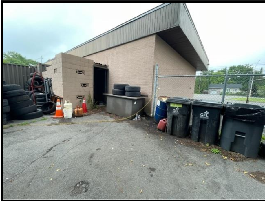
Photograph 7: View of the exterior south wall on the eastern side of the Phase I Property showing the waste oil AST (with 4 tires stacked on top of it).
