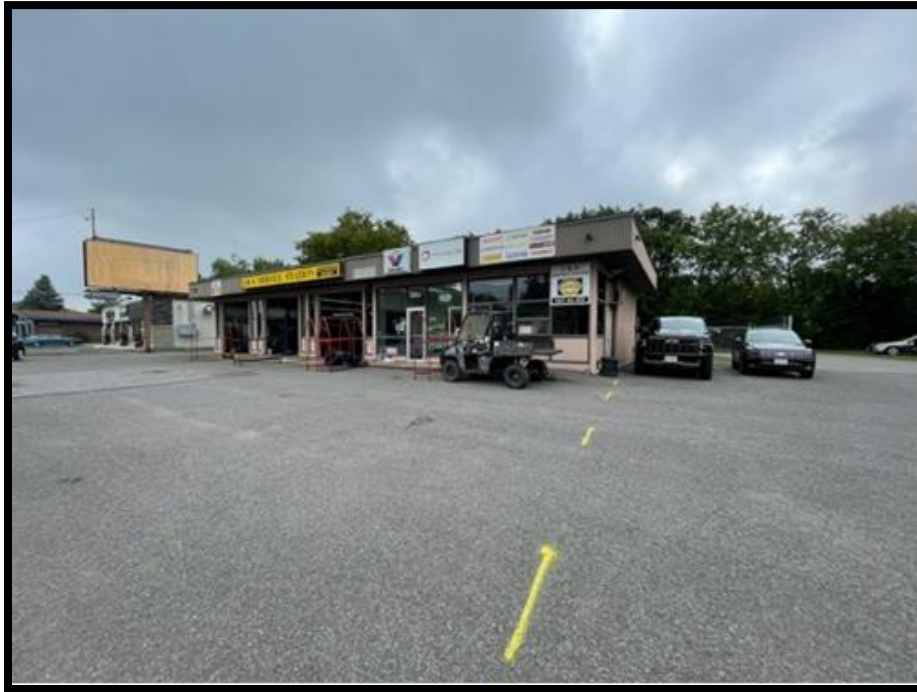
Photograph 1: View of the Phase I Property, facing south from Innes Road.
