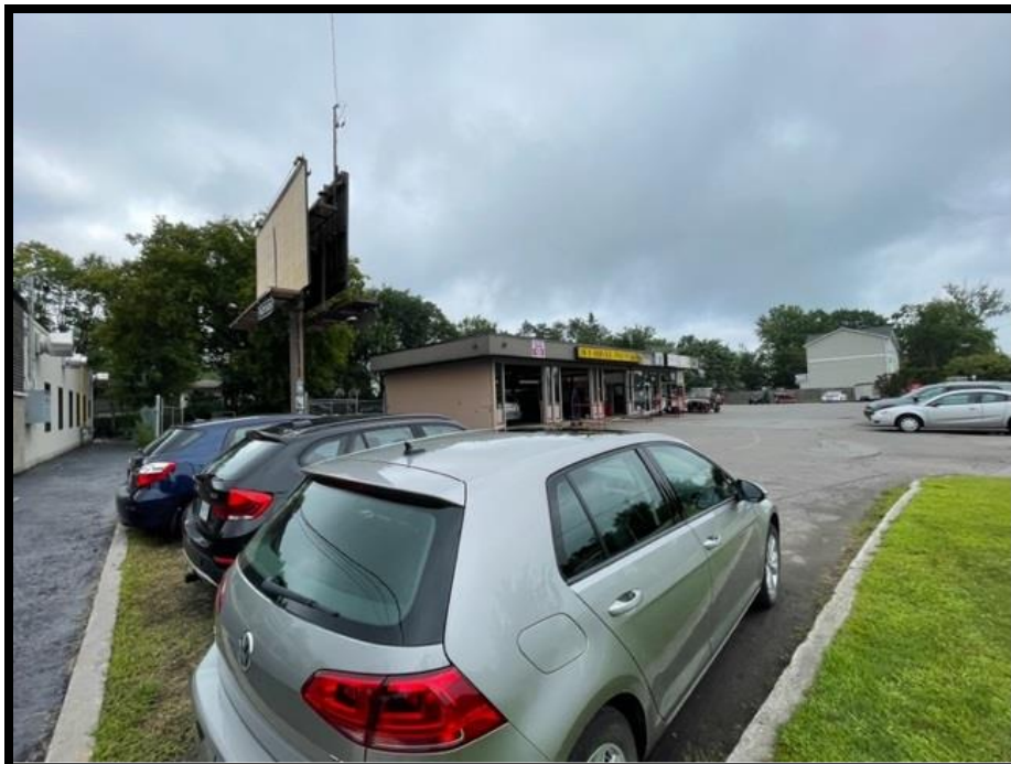
Photograph 2: View of the northeastern side of the Phase I Property, facing southwest.
