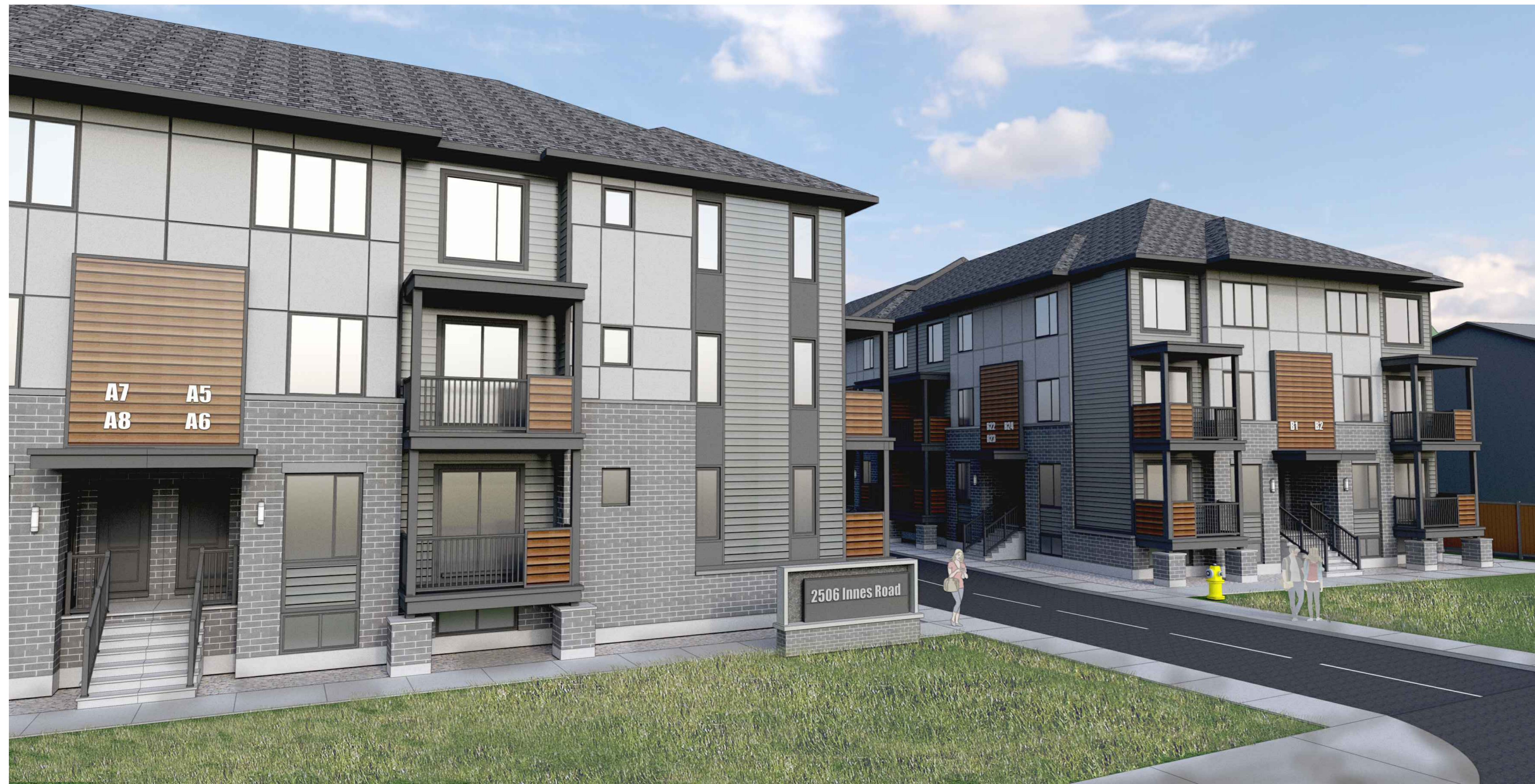
01 | SITE ACCESS VIEW
