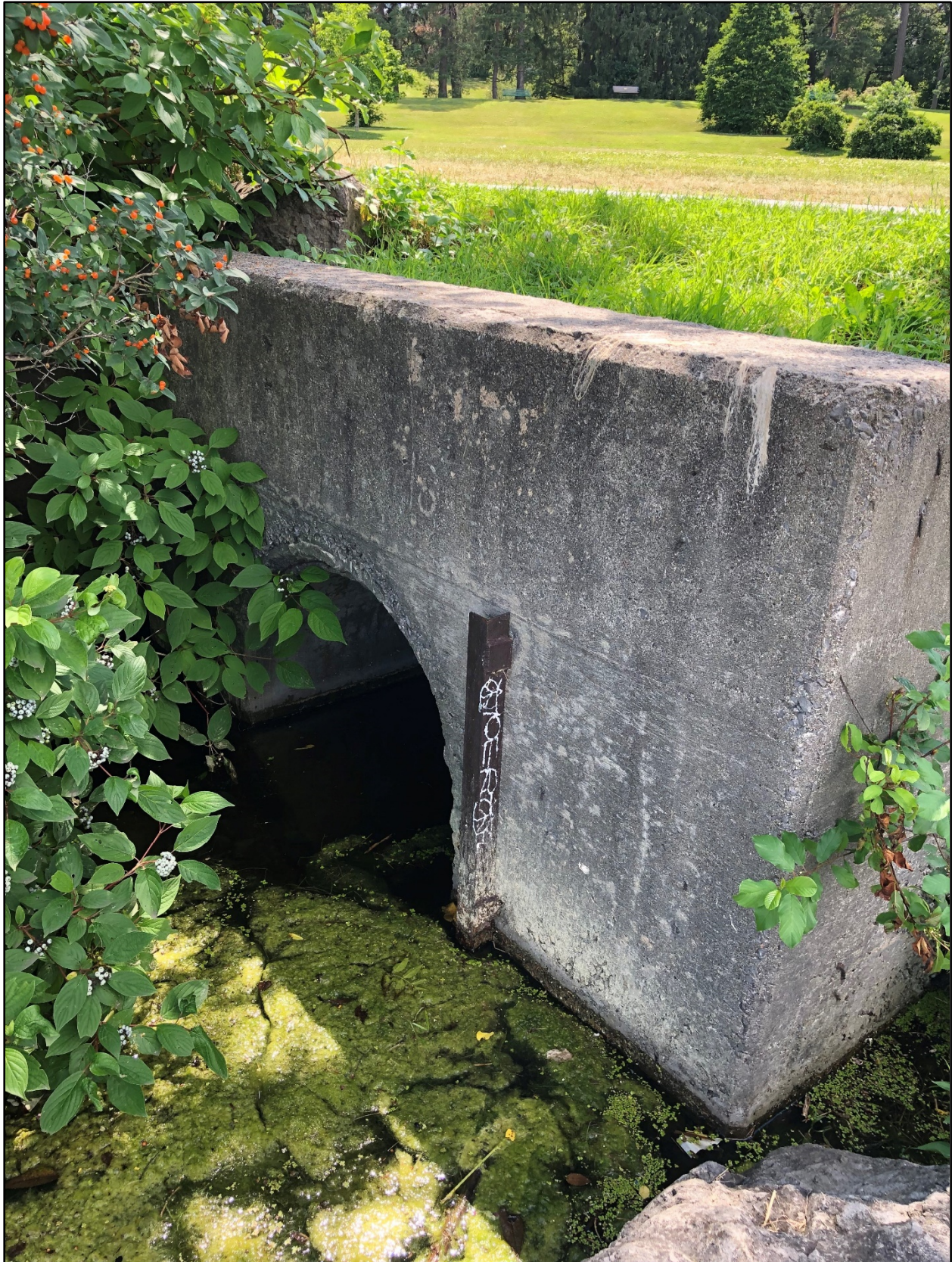
Figure 3: Dow's Lake Outfall - July 2022
