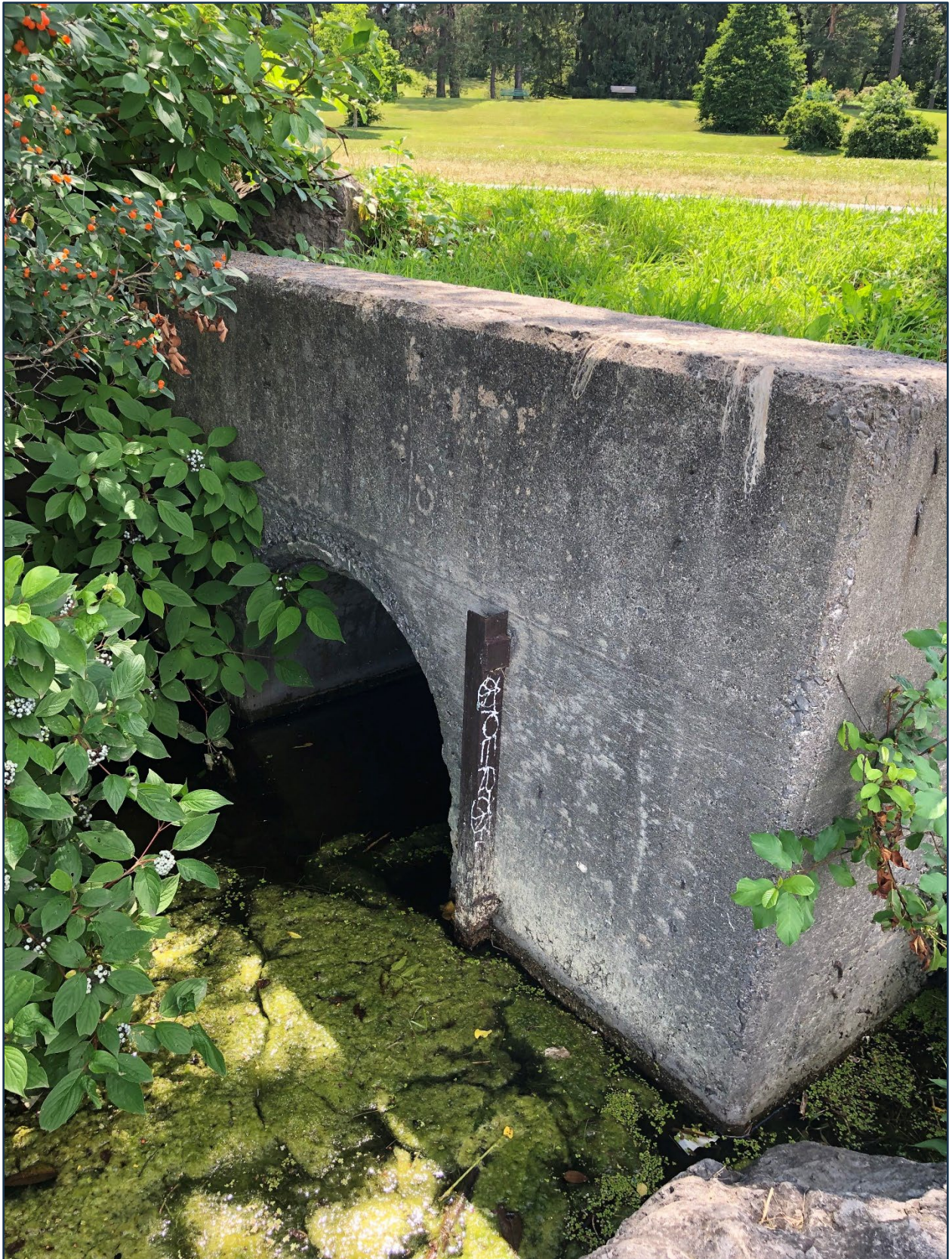
Figure 3-4: Dow's Lake Outfall - July 2022
