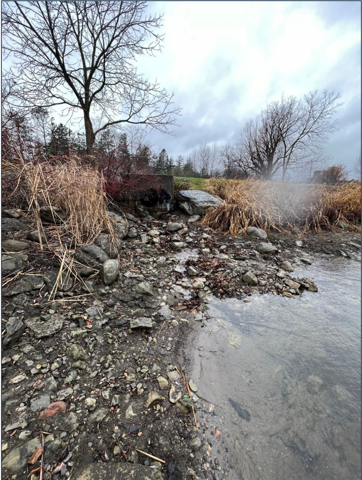
Figure 3-6: Dow's Lake Outfall – December 2022
