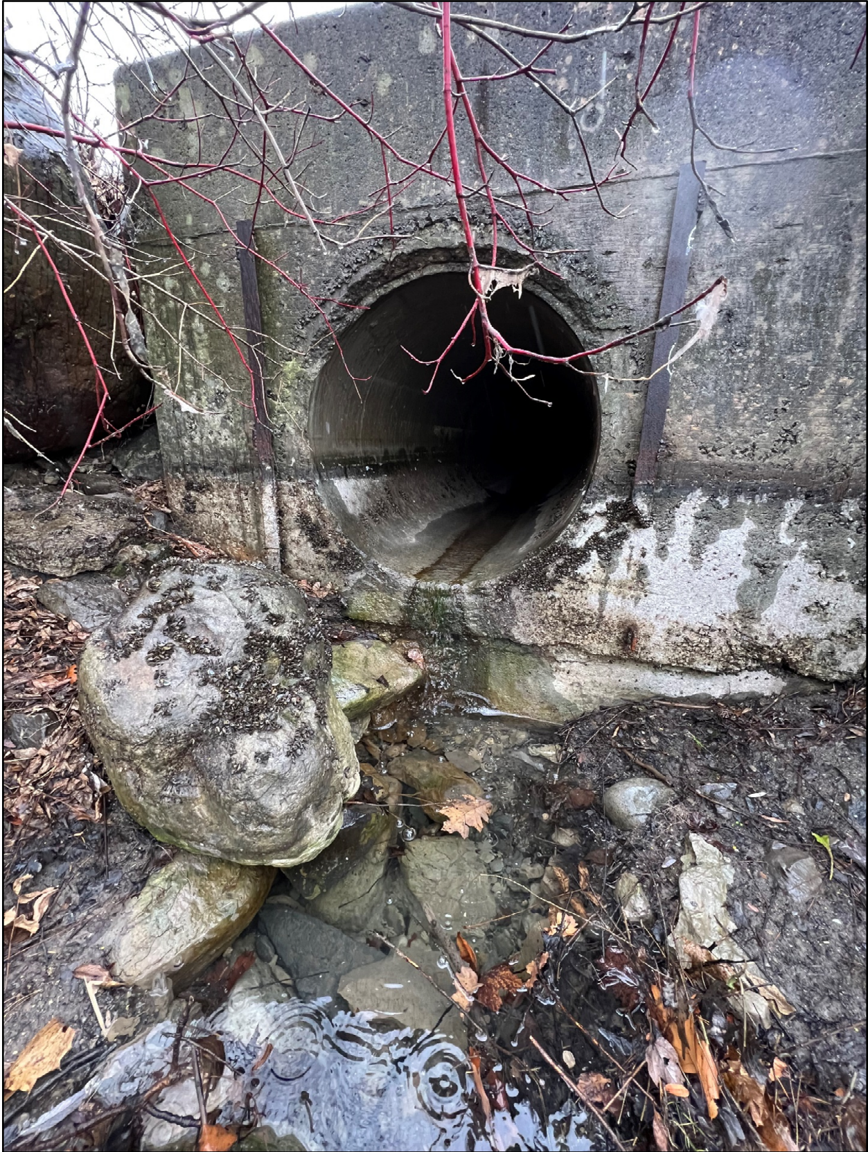
Figure 4: Dow's Lake Outfall – December 2022
