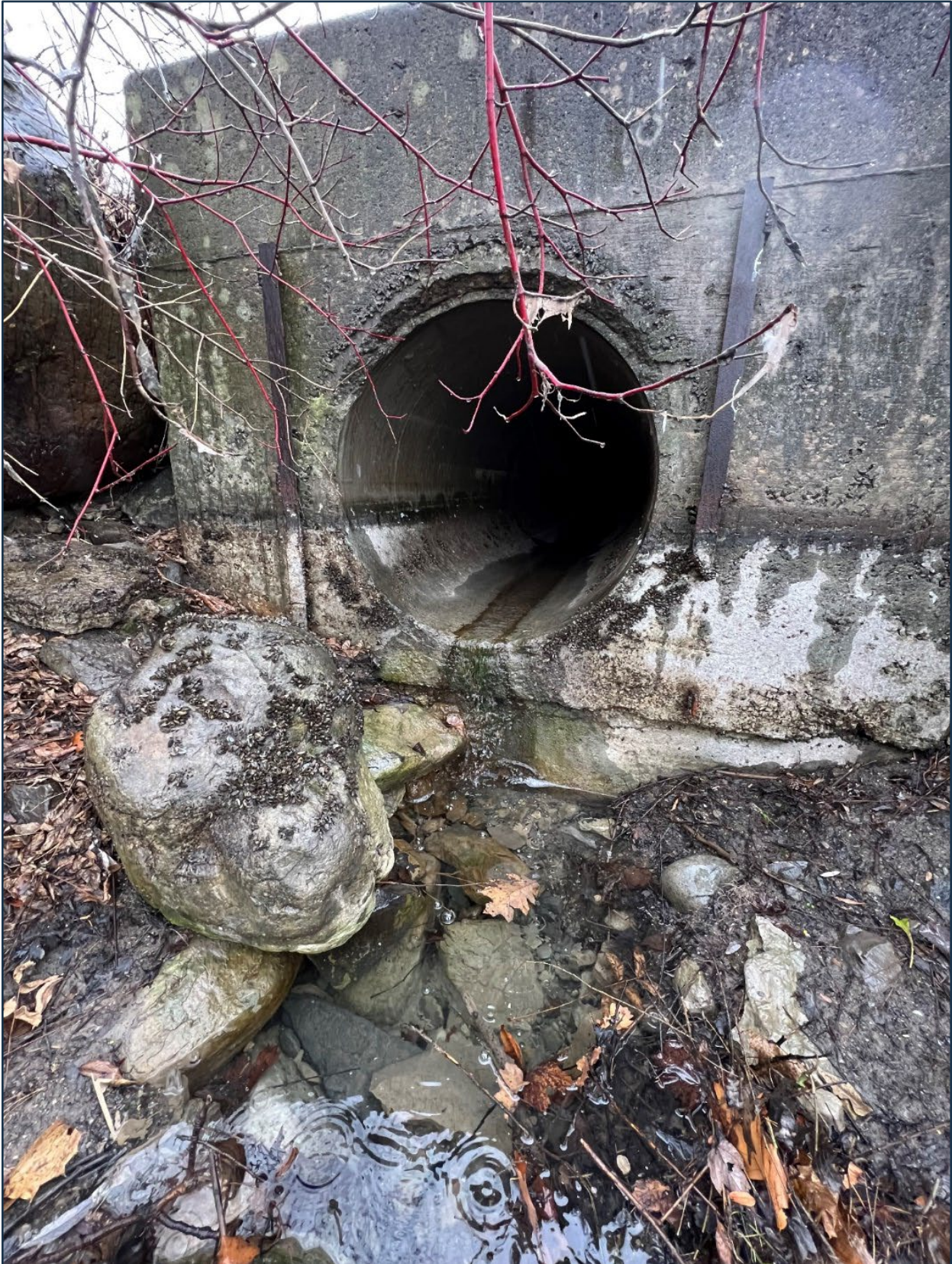
Figure 3-5: Dow's Lake Outfall – December 2022
