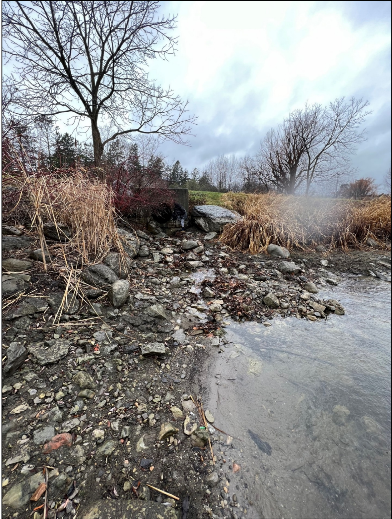
Figure 5: Dow's Lake Outfall – December 2022
