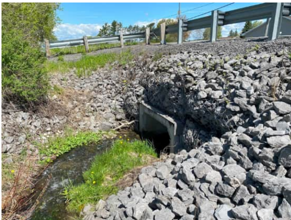
PICTURE 5: Large Box Culvert Crossing Carp Road 1.2km From Site - Facing North
