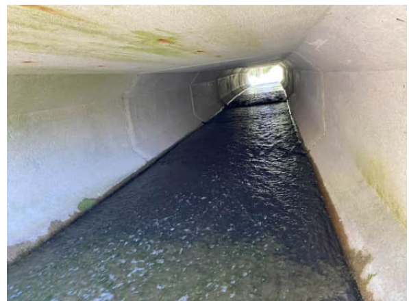
PICTURE 6: Box Culvert Interior in Good Condition - Facing Northeast
