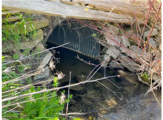
PICTURE 2: Farm Access Culvert with Rock End Protection
