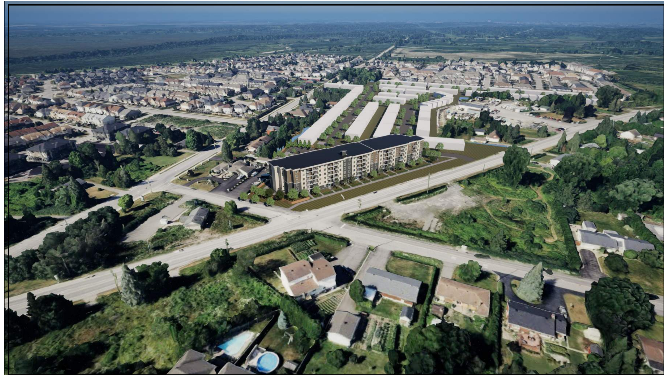
(1) SOUTH - WEST VIEW
