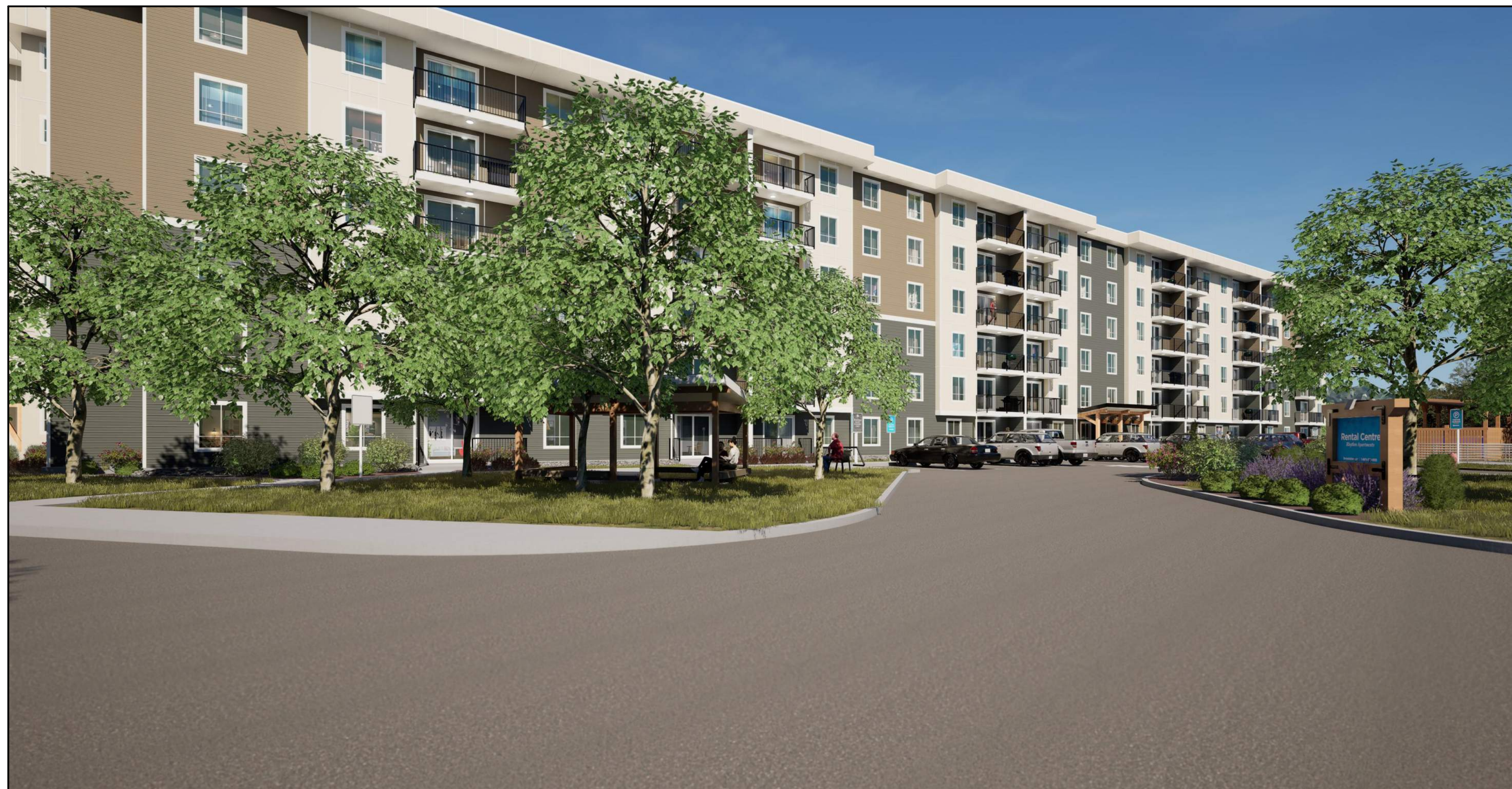
(2) EAST VIEW SITE ENTRANCE
