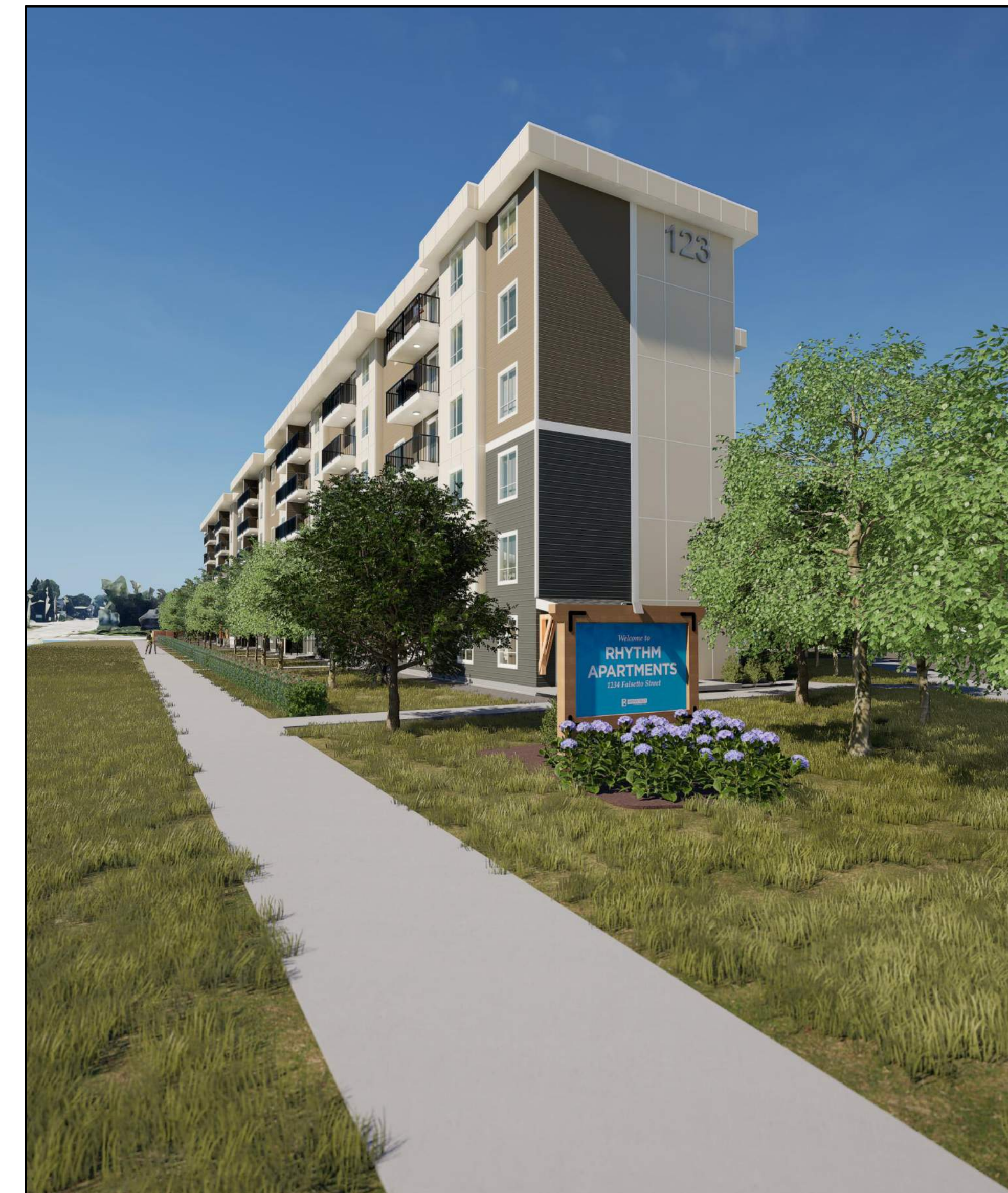
(3) EAST VIEW BUILDING CORNER
