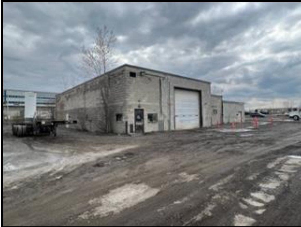
Photograph 2: View of the garage building with maintenance bays on the eastern portion of the Phase I Property.
