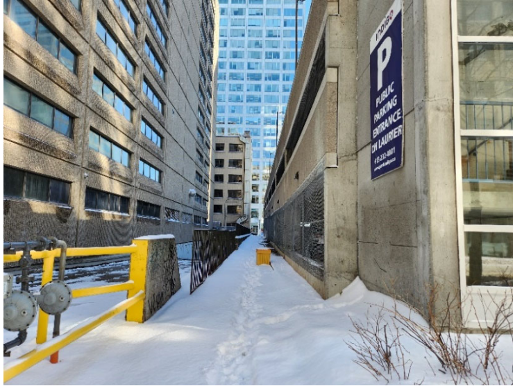
Photo 3 - View of the east side of the garage, looking south.
