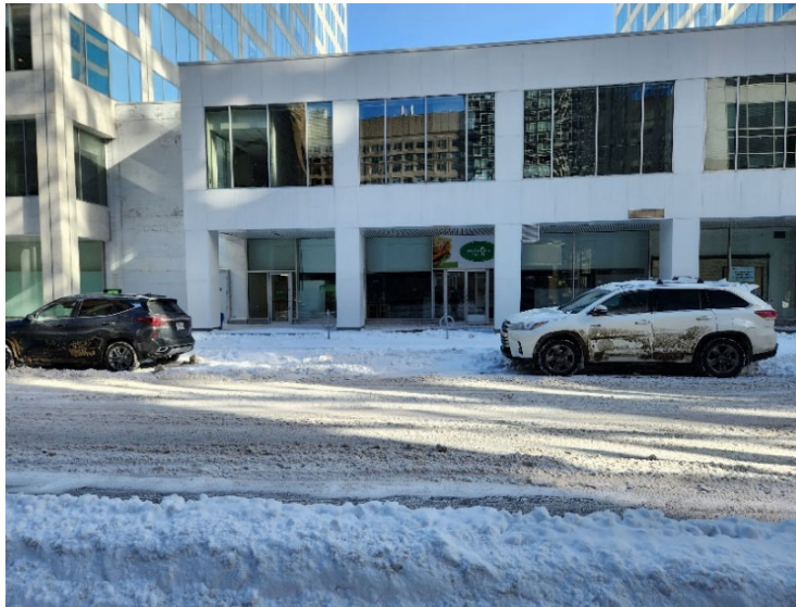
Photo 18 - Looking south from the Property across Laurier Ave
