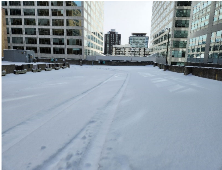
Photo 20 - Upper outdoor level of garage, looking south
