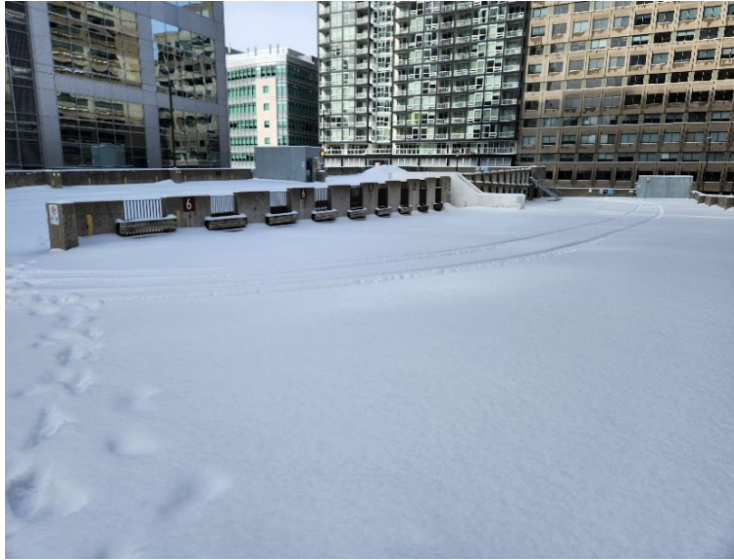
Photo 19 - Upper outdoor level of garage, looking NW
