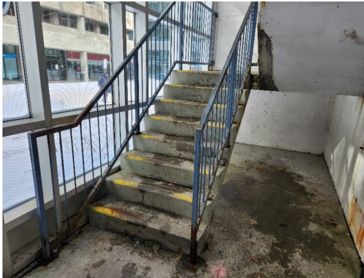
Photo 9 - Stairwell, NE corner of Property
