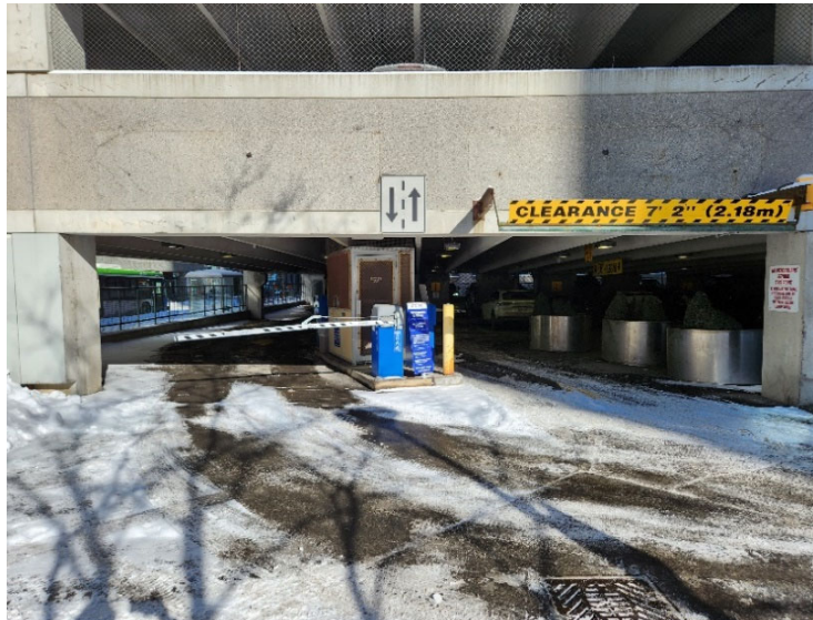
Photo 6 - Parking garage entrance
