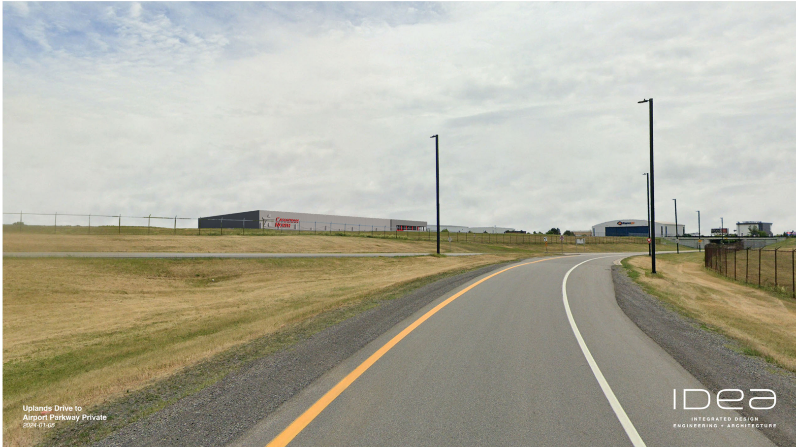
Figure 20 - To Airport Parkway Private looking South
