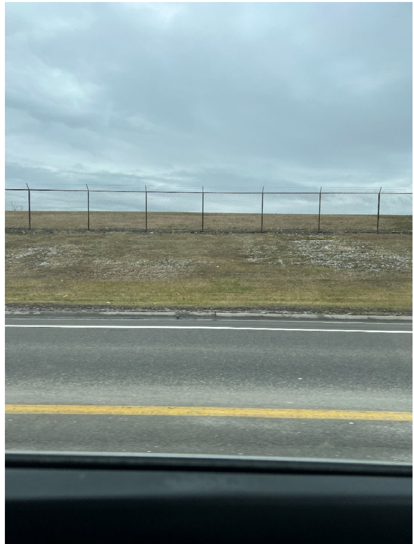
Figure 12 – 10 view looking South from Airport Parkway Private
