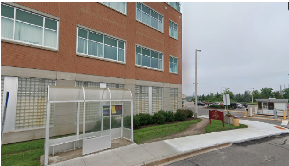
5. View of SE corner of site and bus stop
