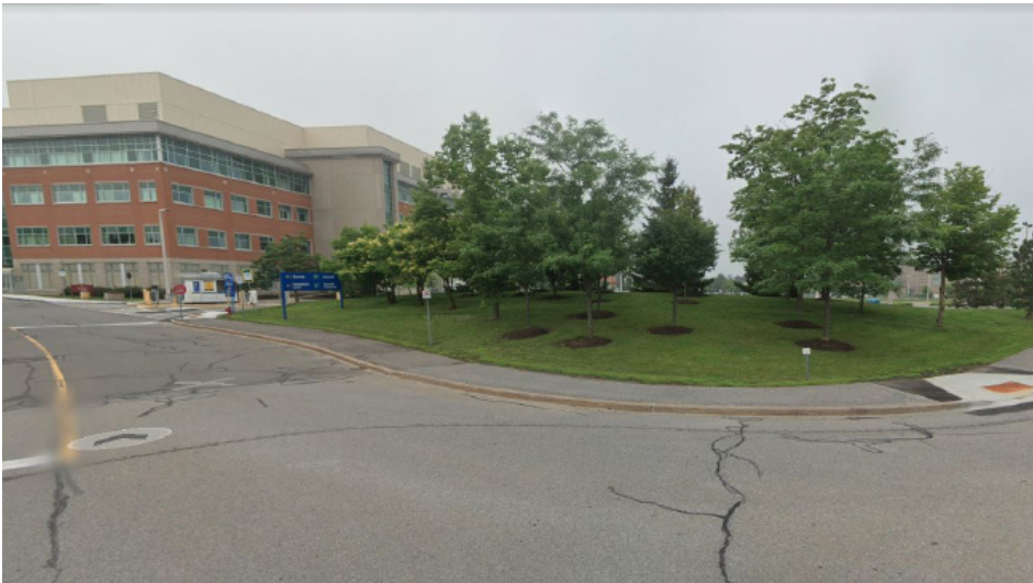
4. View of NE corner of site from Ring Road
