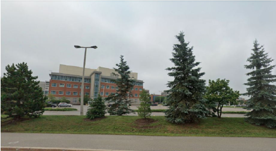
3. View of N face of RGN from Ring Road
