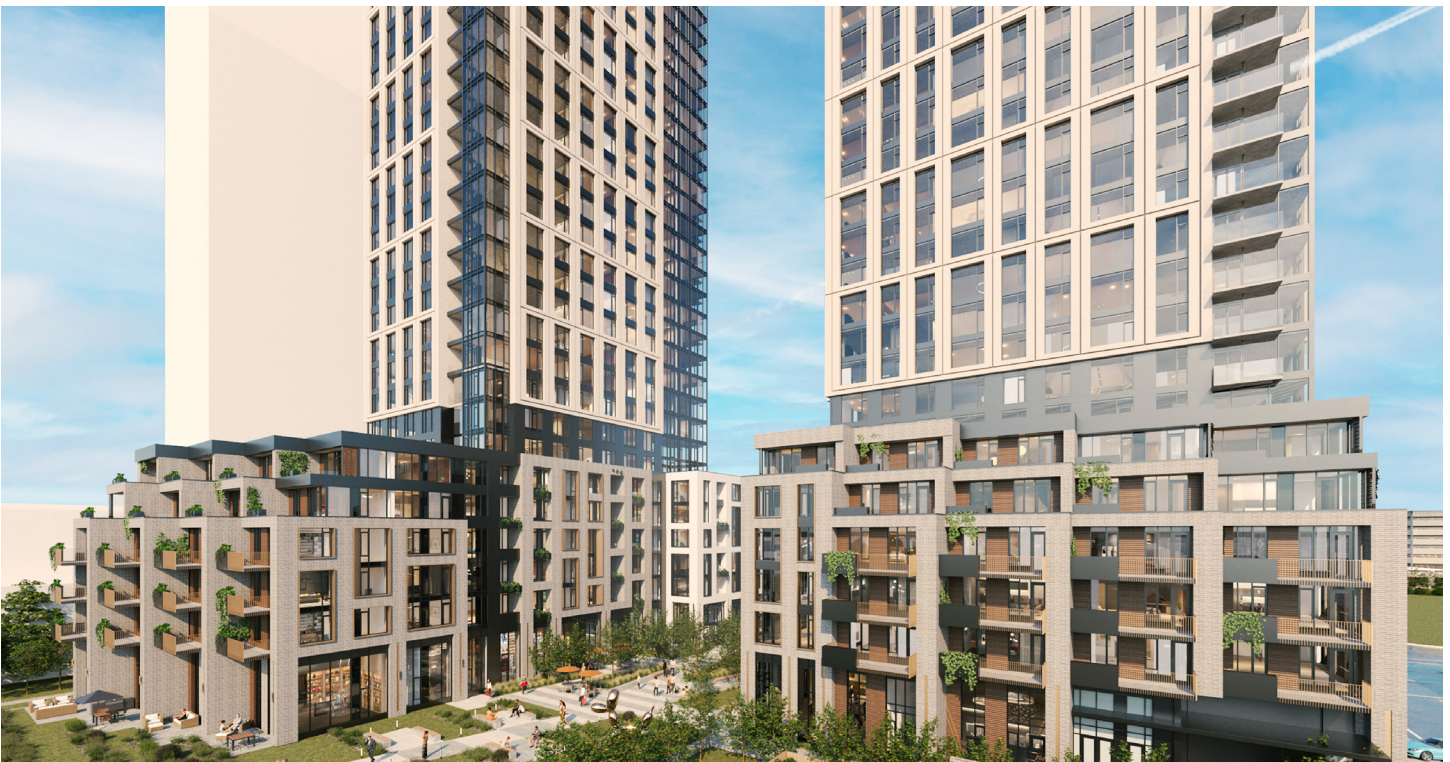
Figure 17.0 - View looking North-West, West building podium terraces.
