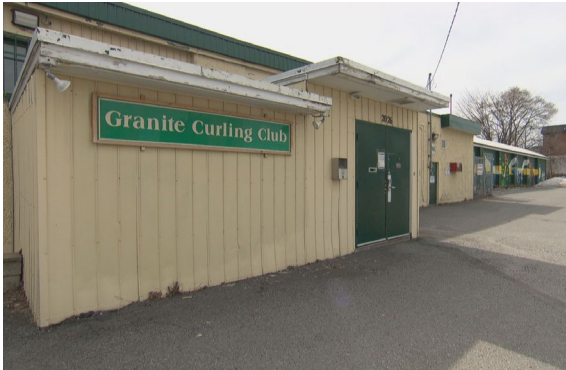
Figure 4.0 - Existing Granite Curling Club, 2026 Scott Street.
