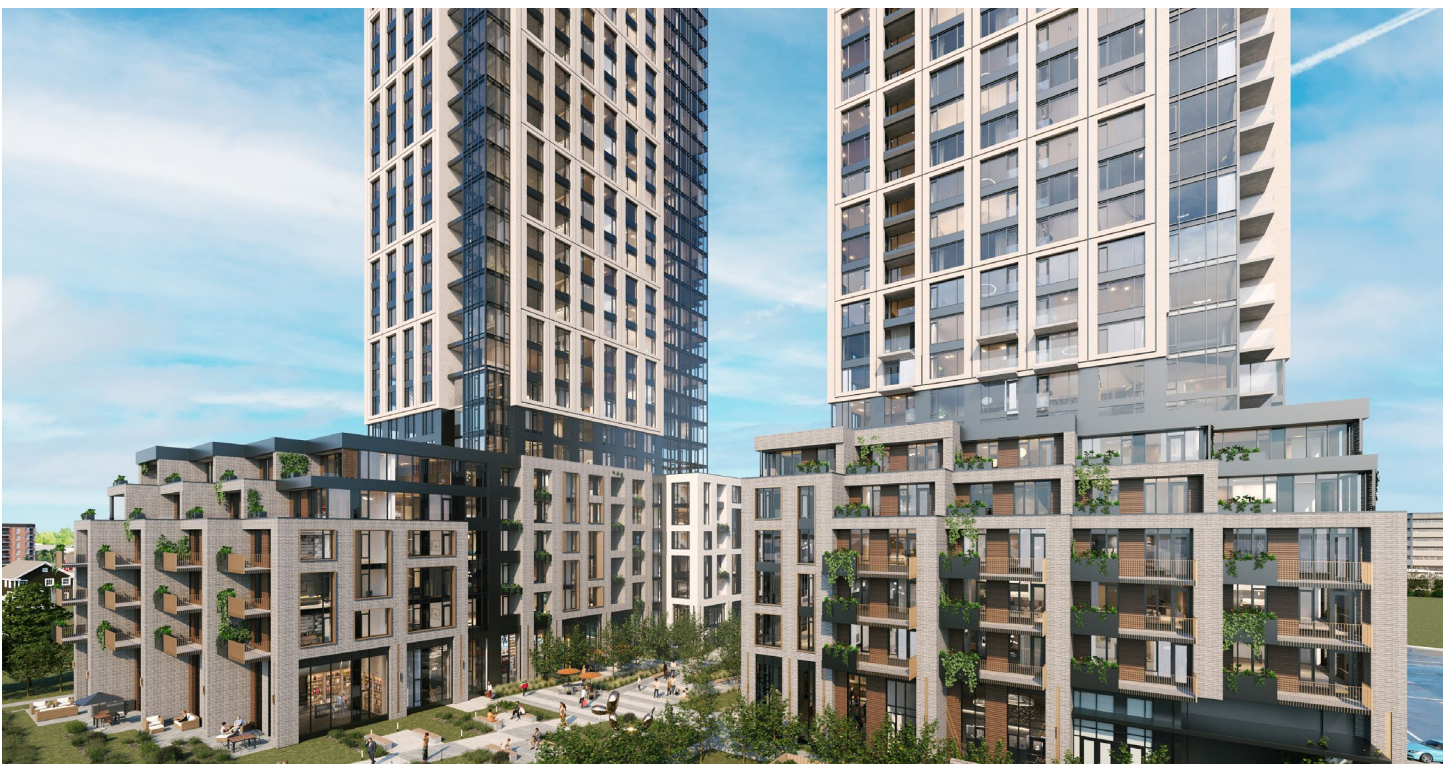
Figure 17.0 - View looking North-West, West building podium terraces.
