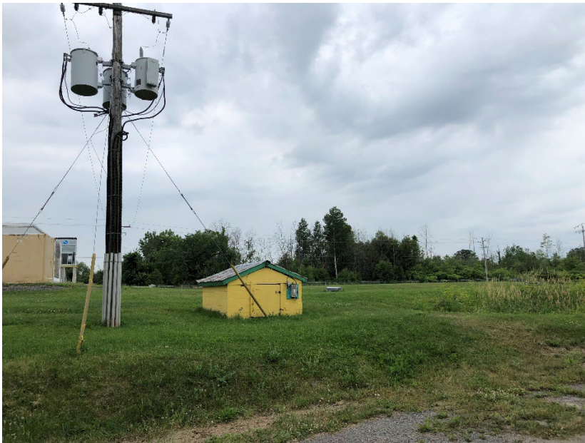
Photo 1 - View of drilled water well TW-1 and pump shed/building.
