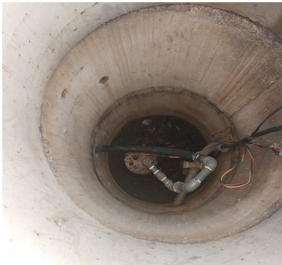
Photo 4 - Interior view of well pit of drilled water well M-1.
