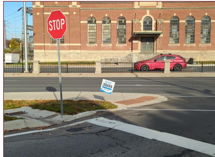
Photograph 8: Power station at 1275 Carling Avenue
