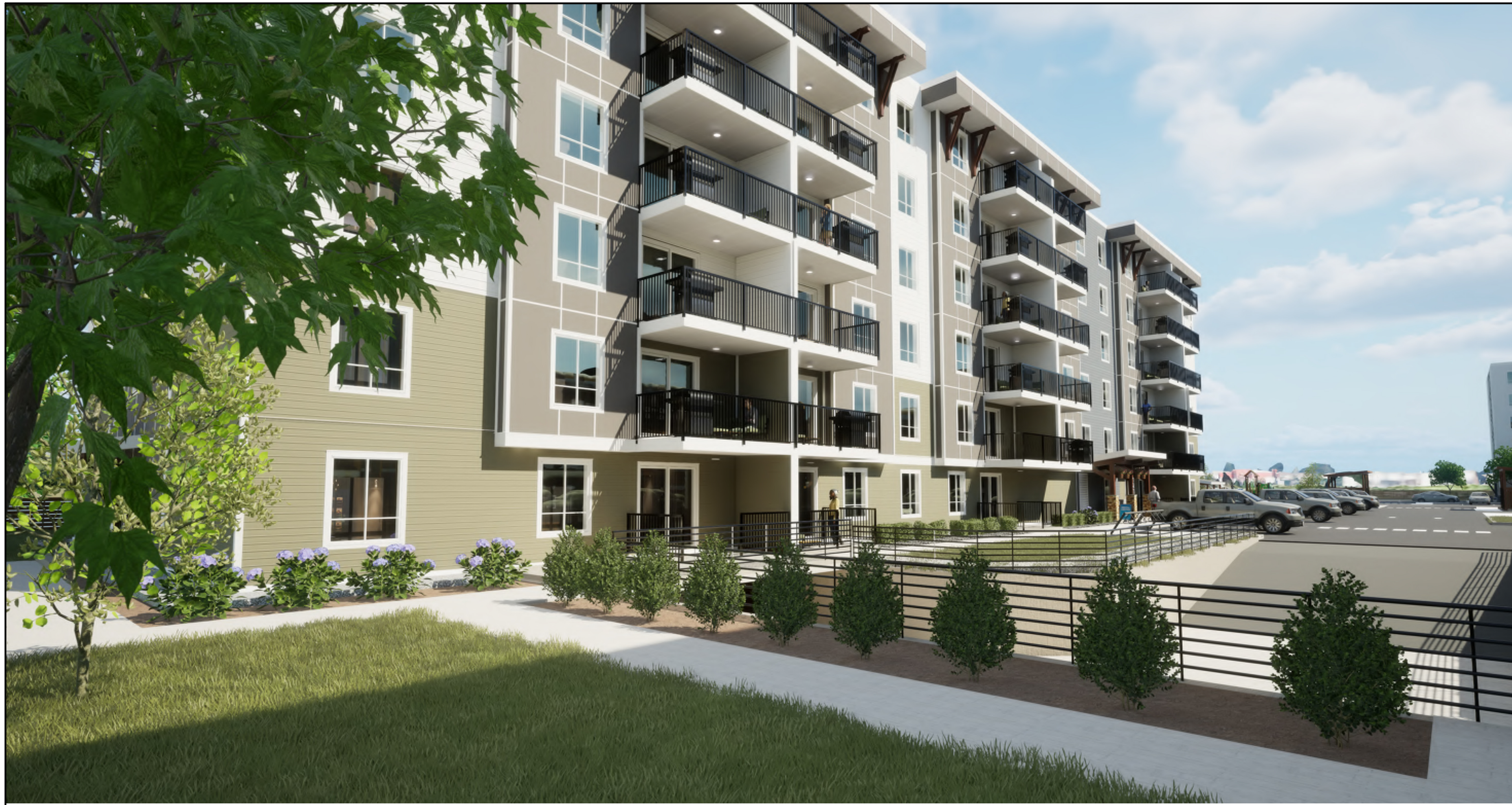
(1) BUILDING D - NORTH VIEW
