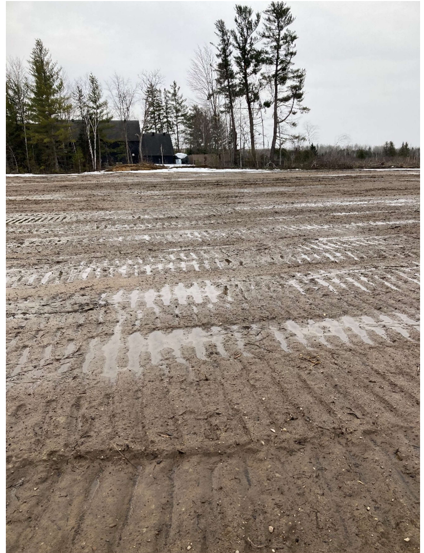
Photograph 4: Overview of 151 Wescar (looking southeast)
