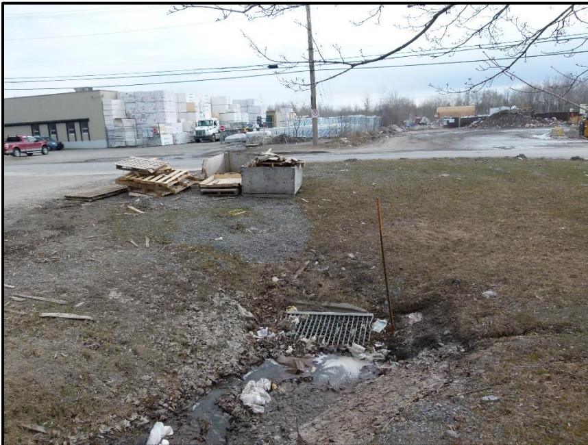
Photograph 2: Looking downstream at the catch basin at Sheffield Road (April 12 th , 2023).
