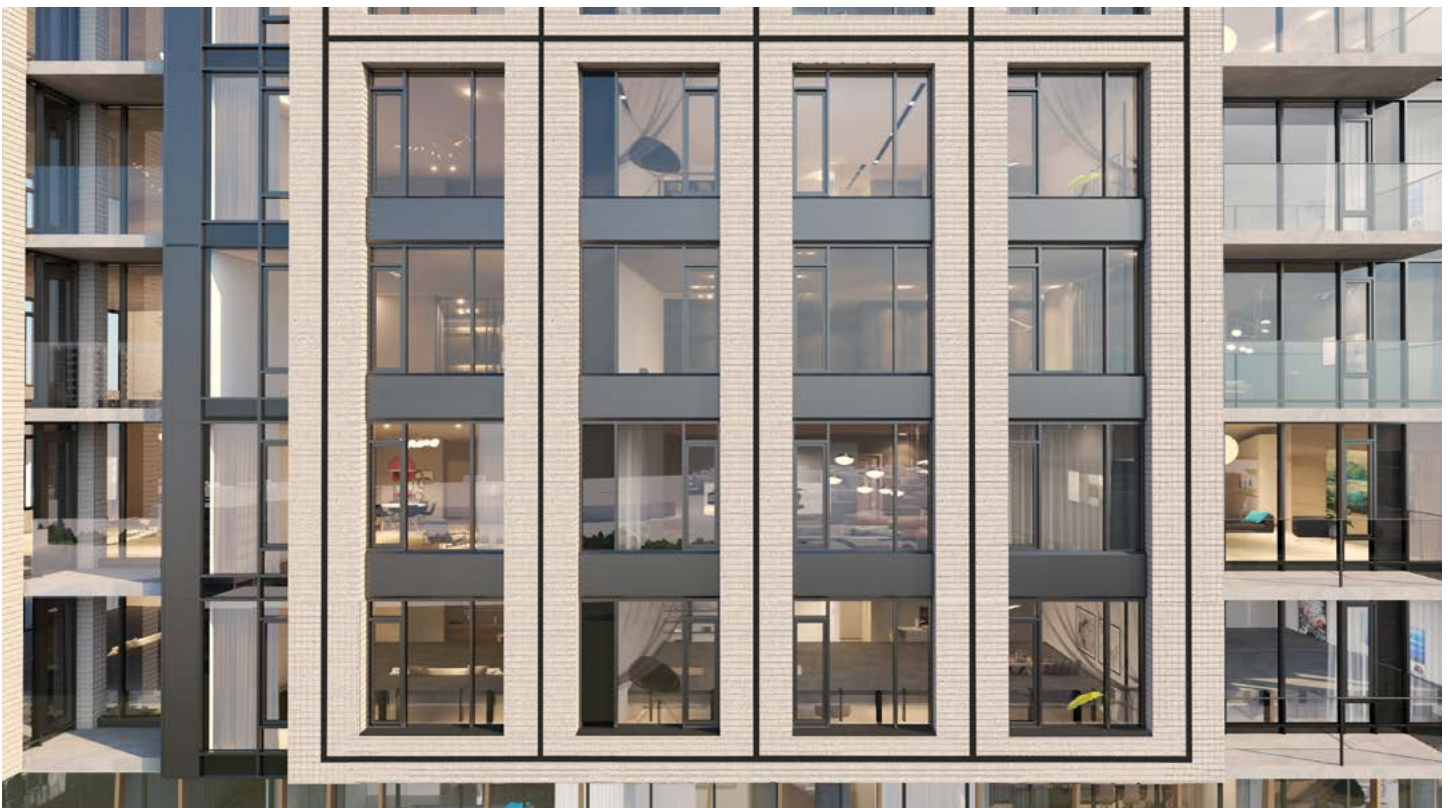
Figure 20.0 - Proposed pre-cast panels on the tower portion of both the East and West buildings.
