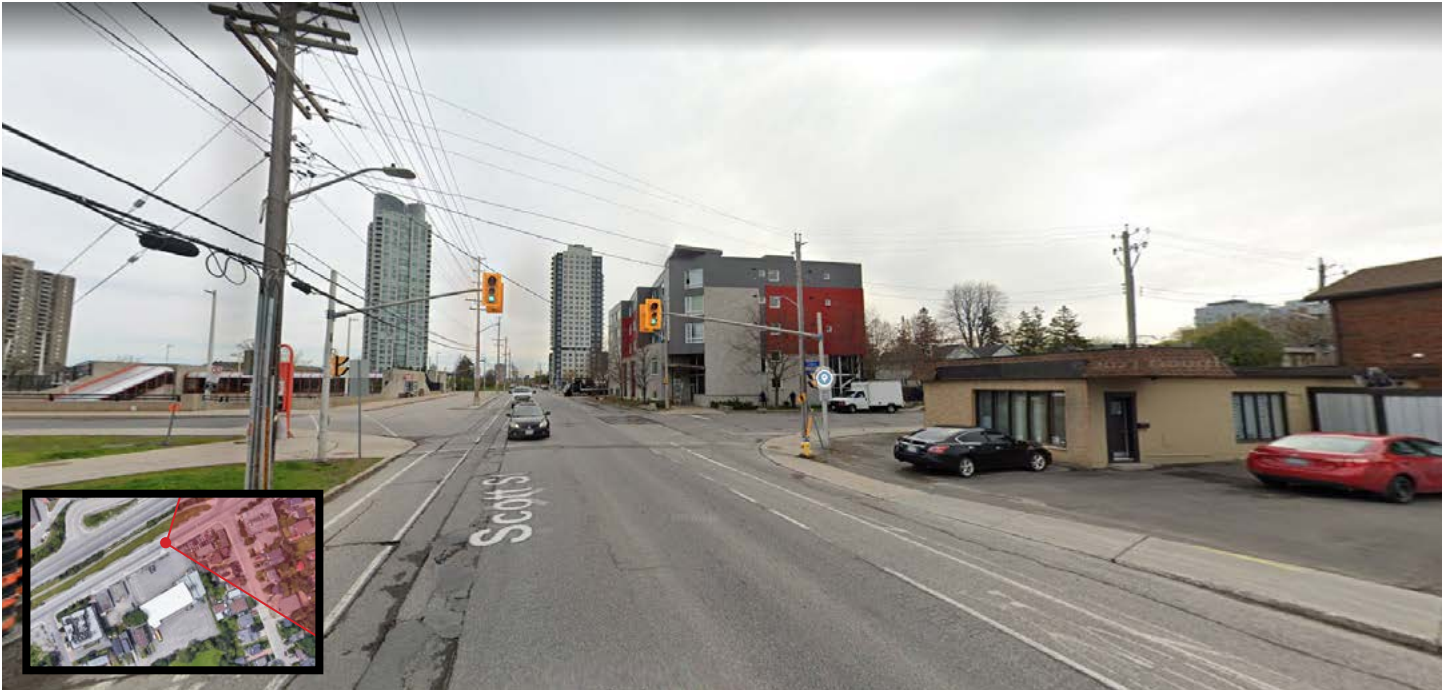
Figure 7.0 - Existing Site Conditions, View East along Scott Street.
