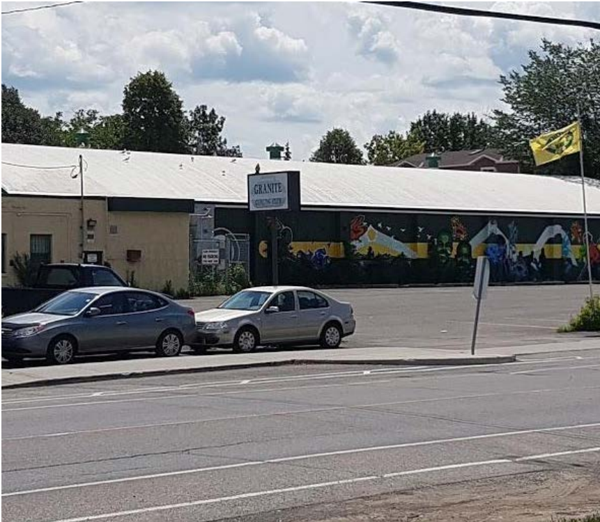
Figure 3.0 - Existing Granite Curling Club, 2026 Scott Street.
