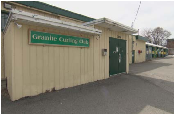
Figure 4.0 - Existing Granite Curling Club, 2026 Scott Street.
