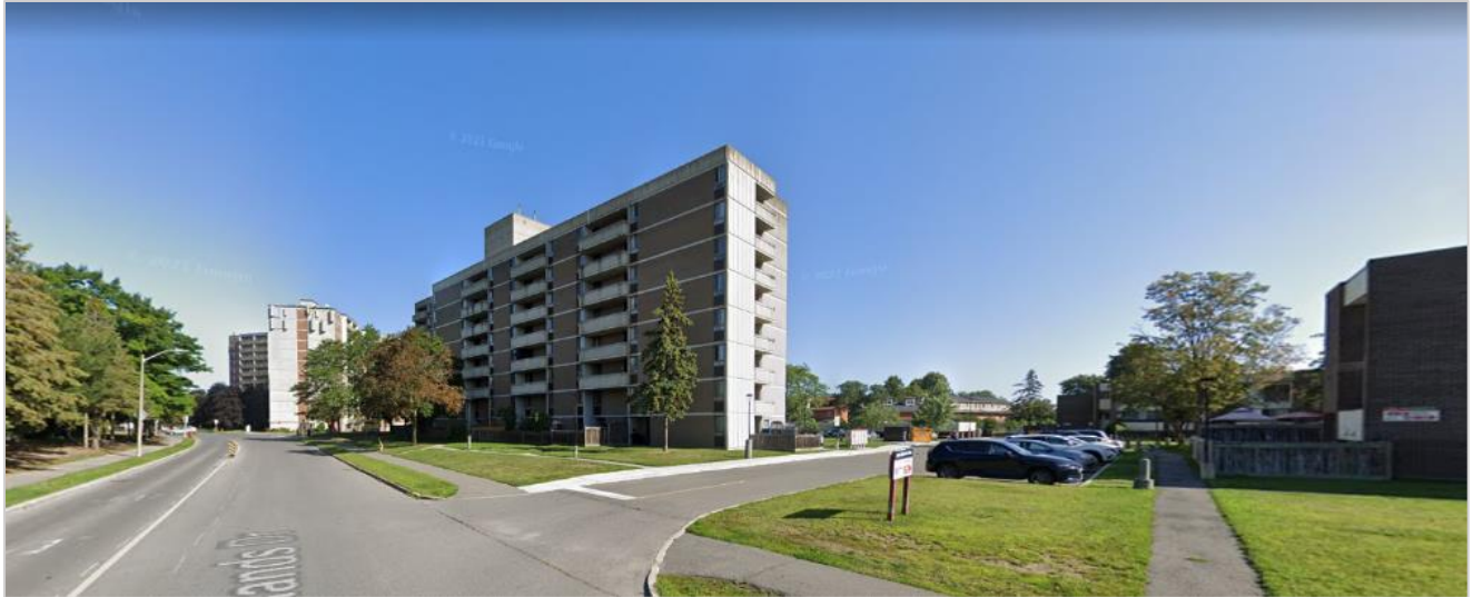
Figure 8: Mid & High Rise Residential, Northwest of Subject Land (Source: Google StreetView)
