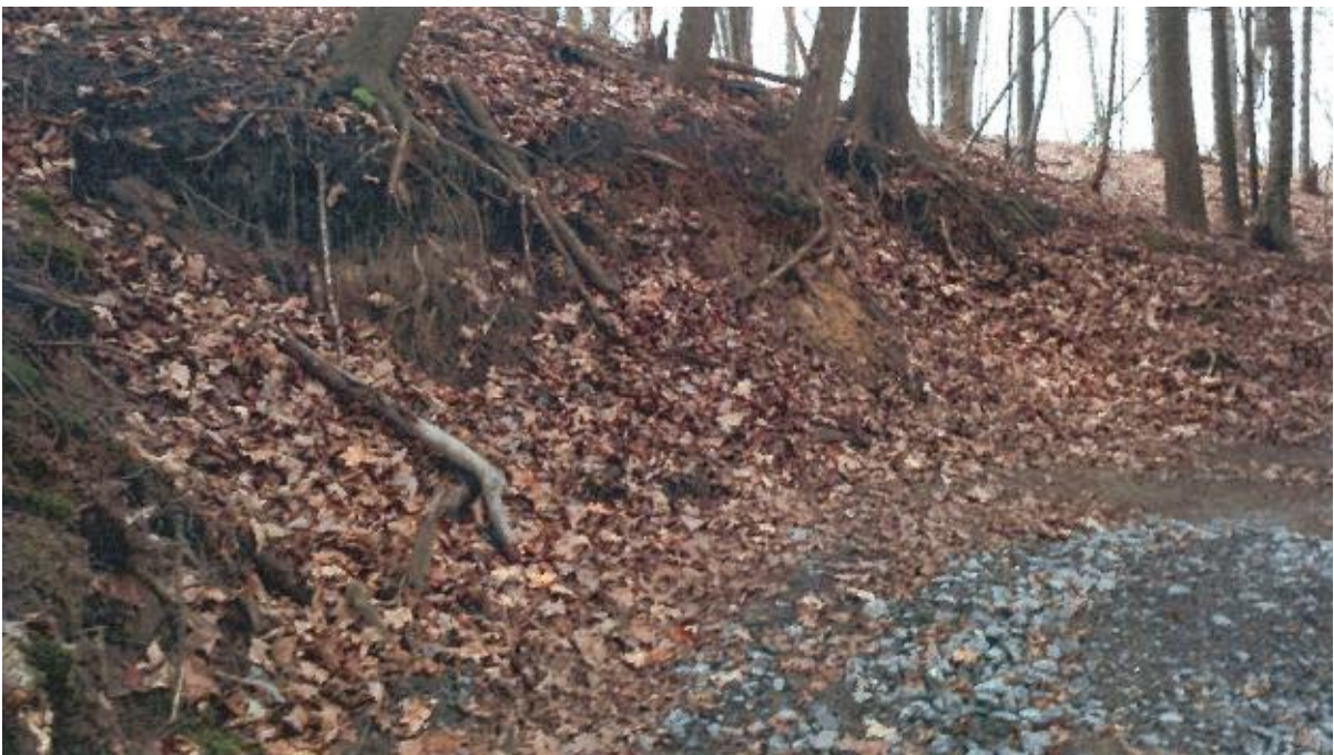
Photo No. 12 – Erosion of slope uphill of pathway.
