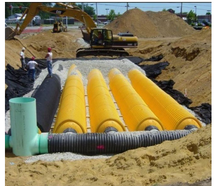
Looking down the Isolator Row PLUS from the manhole opening, ADS PLUS Fabric is shown between the chamber and stone base.
