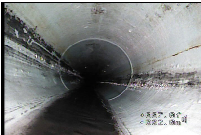
Figure#5: A view to the 30% water level at 6.6 meters from the top of MHSA1.
