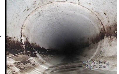
Figure#10: A view to the left line deviation and water mark shown pipe at full capacity at 15.8 meters from the top
