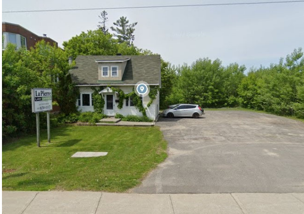
Photo 1: Existing structure at 2663 Innes Road
