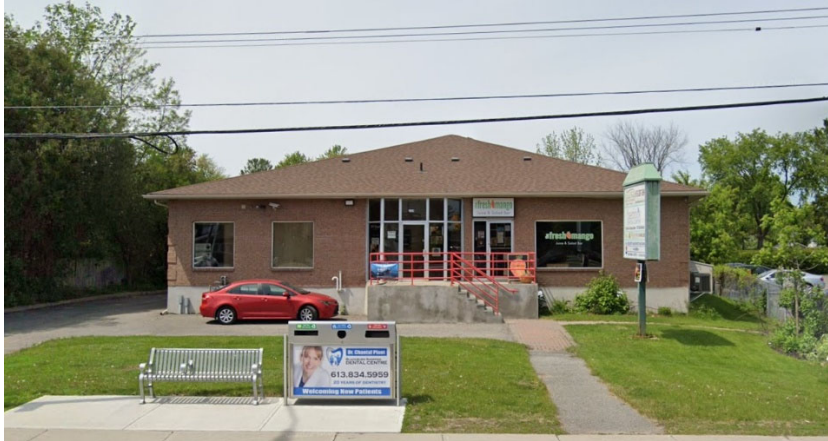
Photo 14: Commercial Multi-Office space abutting Innes Road
