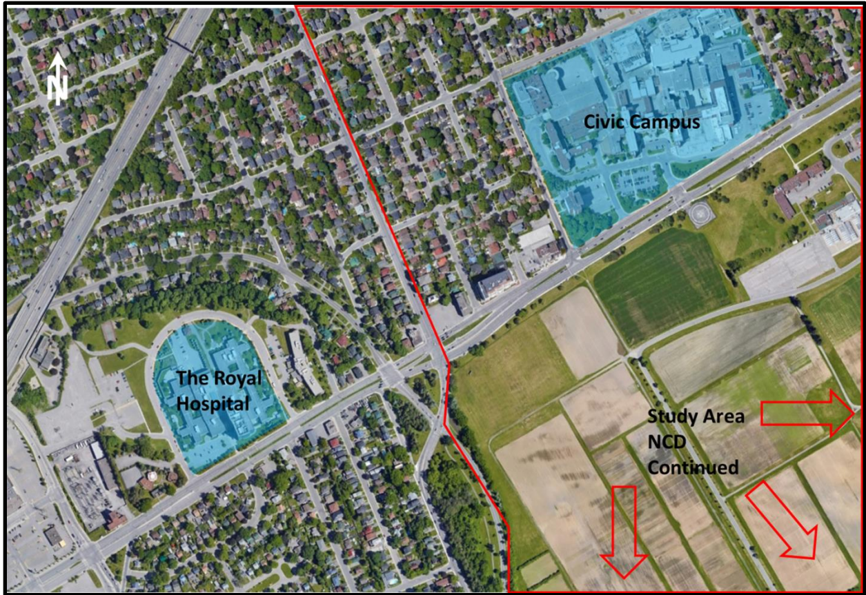
Figure 4: The Royal Hospital Site
