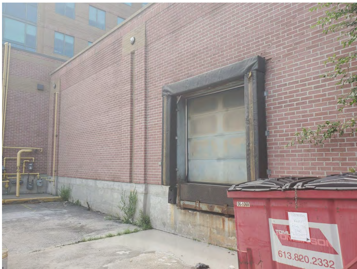
Photograph 3: Site, south side.
