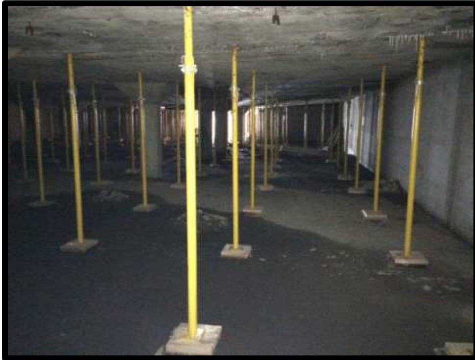
Photograph 3: View of the interior of the lower level of the parking structure. Facing west from the eastern end of the structure.
