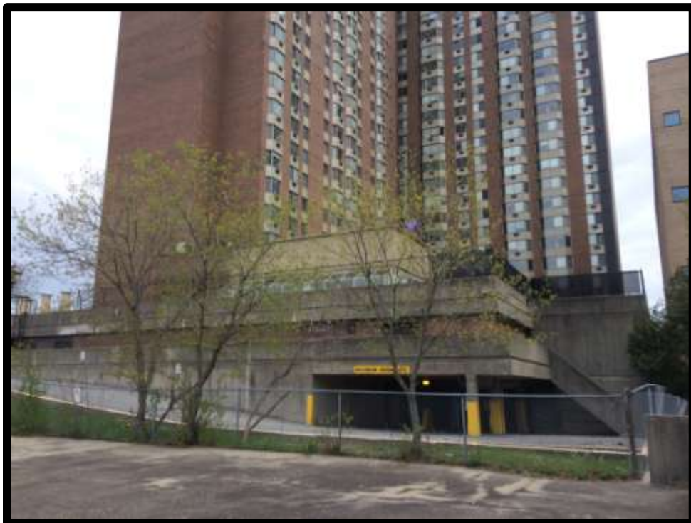
Photograph 8: View of neighbouring property to the south, occupied by a residential apartment tower with an underground parking structure.
