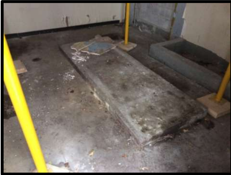
Photograph 1: View of former generator room. The concrete slab and berm are evidence of the former generator and tank locations. Concrete was observed to be in good condition with minimal staining.
