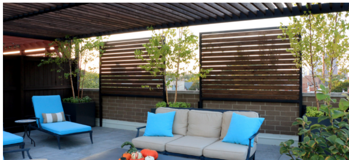
Wooden slat privacy screens with metal frame
