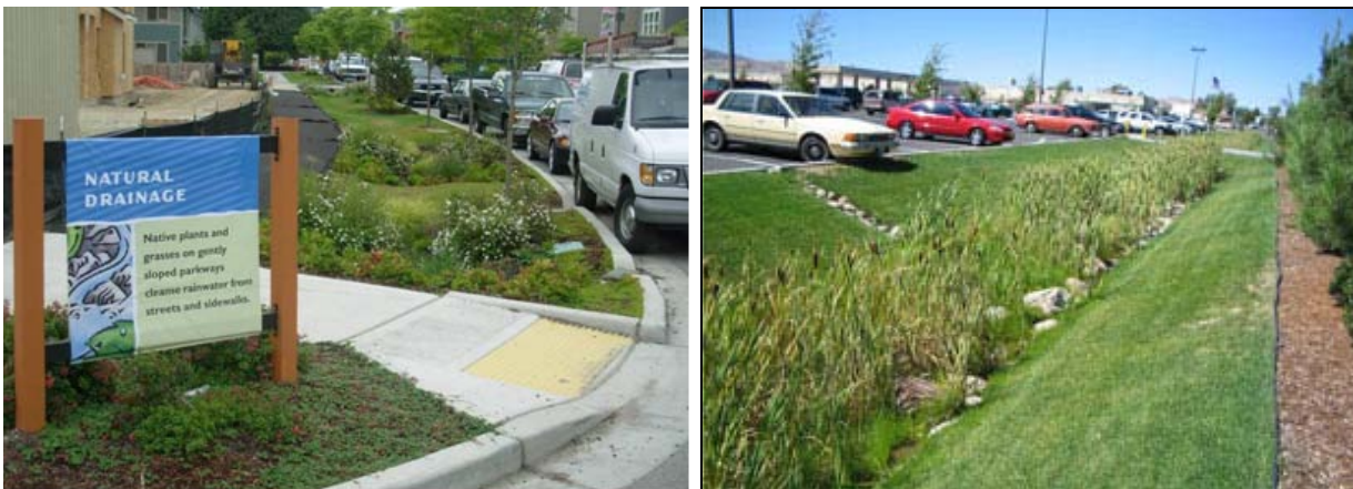
Figure 4.8.1 Enhanced grass swales can be applied in road rights-of-way or along parking lots
