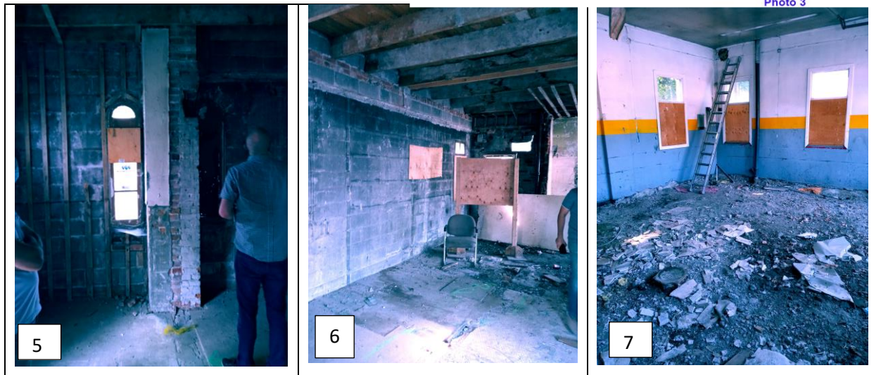
Figure 19: Interior views; 5. Looking towards the east wall with round headed windows on either side of the chimney. View 6. And 7. Interior views of transition area and the service bays. Source Commonwealth 2021
