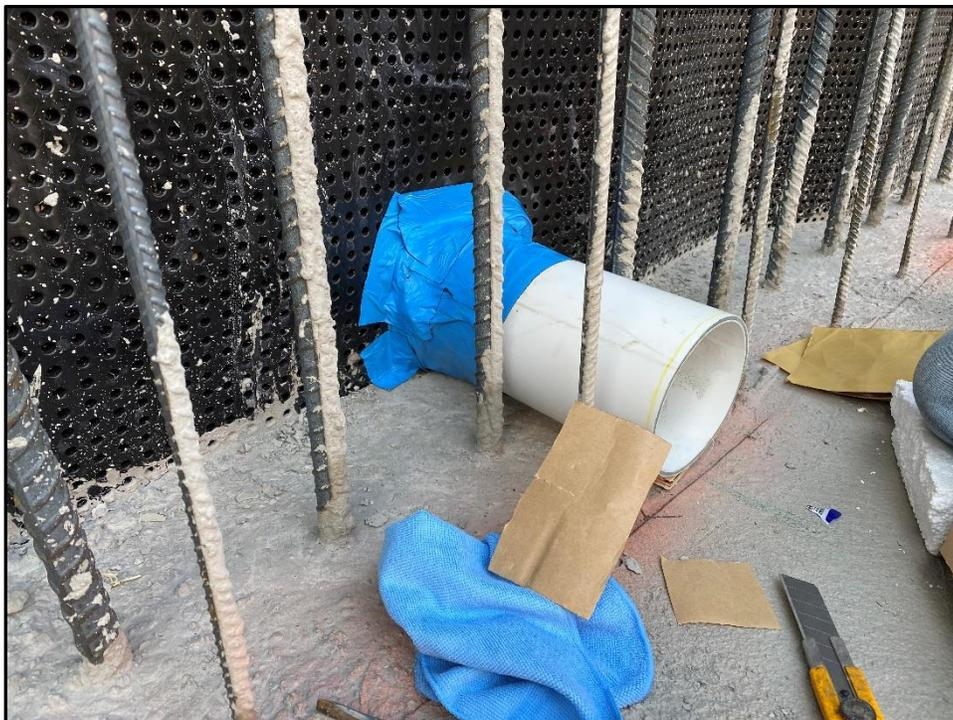
Photo 5 – Step 5: As an additional precaution, it is also recommended that an adhesive tape be placed on the interior outlet end of the drainage sleeve between the temporary form work to further prevent concrete from entering the drainage sleeve during the placement of concrete. Once the temporary form work has been removed, the adhesive tape can be cut away to allow groundwater to have a positive gravity connection to the interior perimeter and underfloor drainage system.
