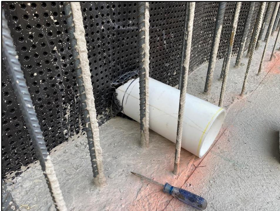
Photo 3 – Step 3: Apply a suitable primer prior to the placement of the adhesive tape such as 3M tape, WP200 BlueSkin or equivalent.
