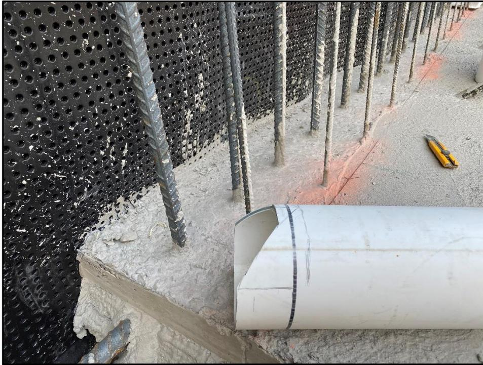
Photo 2 – Step 2: It is recommended that the 150 mm diameter drainage sleeve be installed by carefully cutting an 'X' shaped incision through the composite foundation drainage and inserting the 150 mm diameter drainage sleeve inside the 'X' by pulling the four (4) triangular flaps towards the installer.
