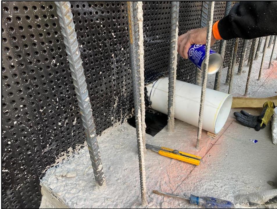
Photo 4 – Step 4: An adhesive such as 3M tape, BlueSkin, or equivalent be utilized to seal the 150 mm drainage sleeve to the composite foundation drainage board to act as a barrier in preventing concrete from blocking connection during the placement of the exterior concrete foundation wall.
