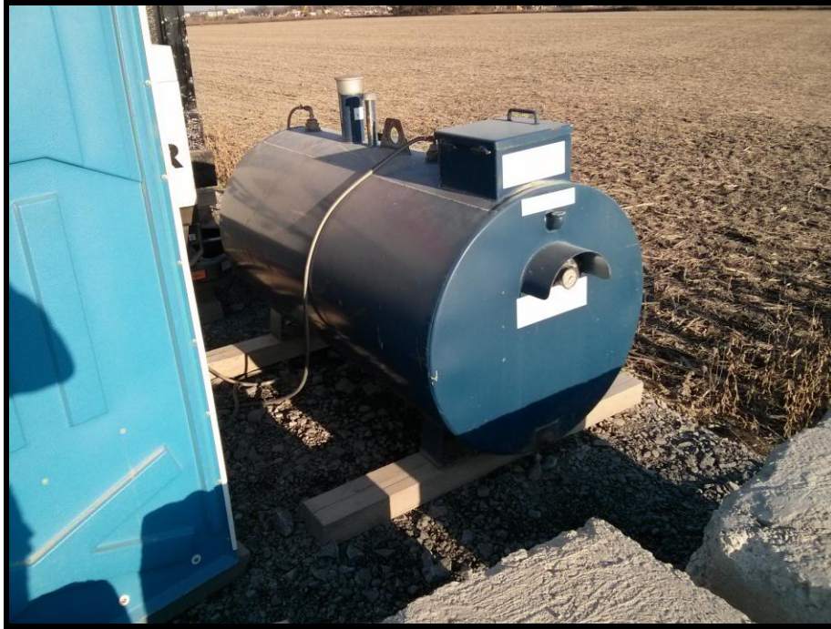
Photograph 3: View of the aboveground storage tank located in the central portion of the property, facing southwest.
