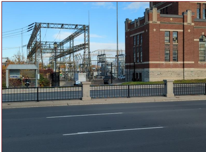
Photograph 7: Power Station at 1275 Carling Avenue.
