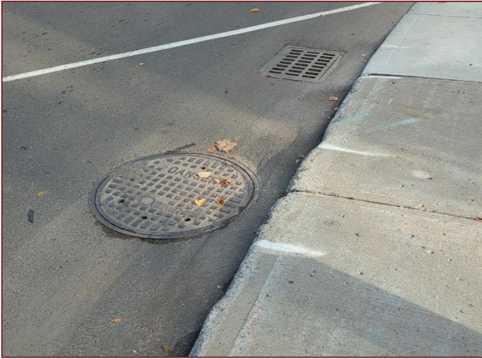
Photograph 9: Storm drain on side of road outside home
