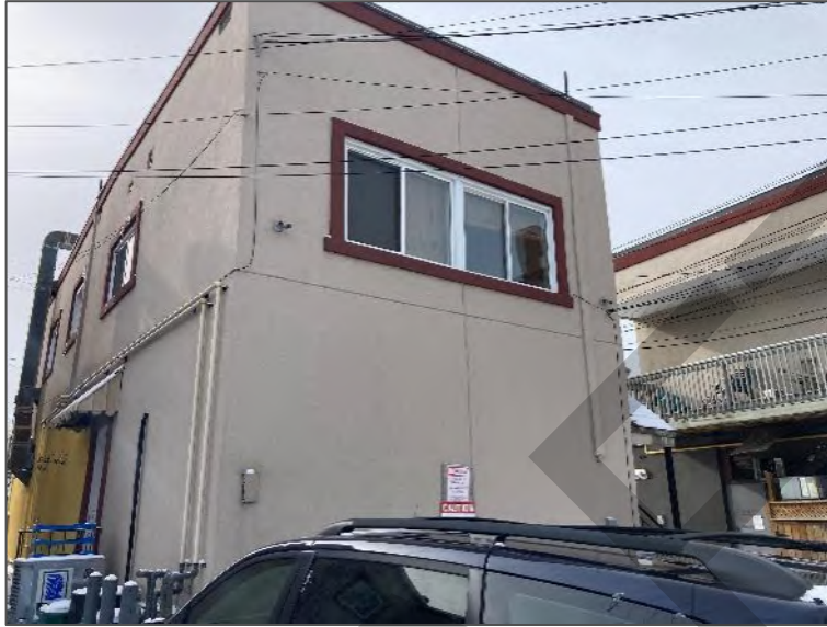
Photo 9 – South elevation of Site Building C, looking north.
