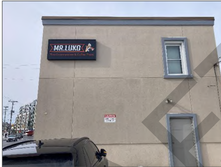
Photo 5 – West elevation of the Site Building B, looking west.
