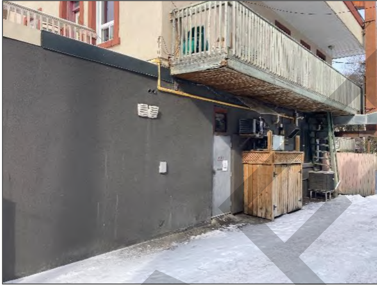
Photo 3 – East elevation of the Site Building A, looking northwest.
