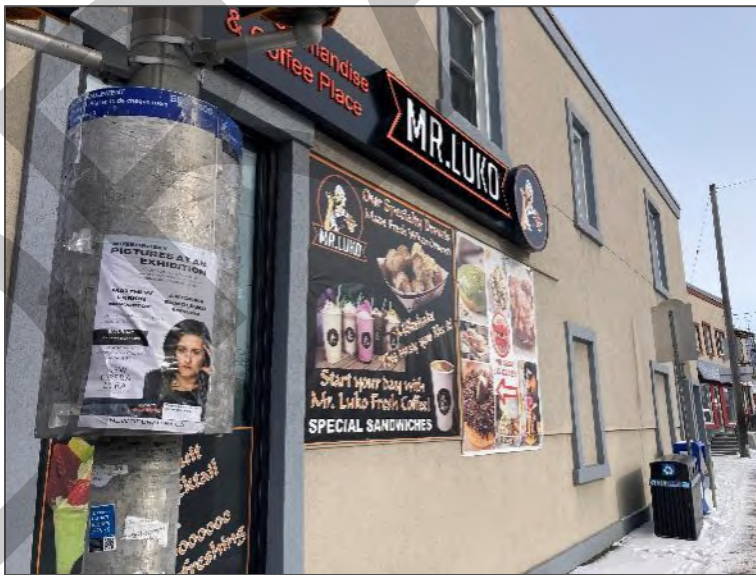
Photo 4 – South elevation of the Site Building B, looking west.
