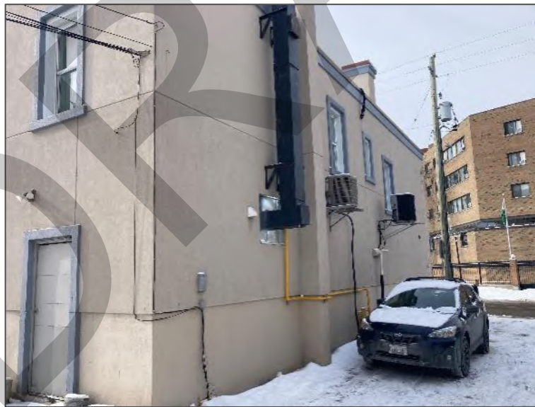
Photo 6 – North elevation of the Site Building B, looking southwest.
