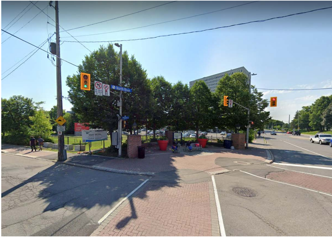
North-West Corner of Property – Facing South-East
