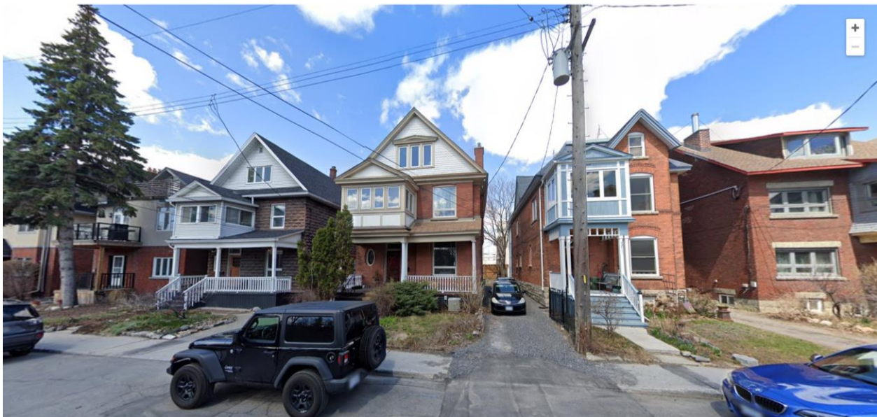
Figure 4: A View of the two 'Registered' properties at 39 and 43 Rosebery Avenue. Neighbouring buildings include the fine example of Boyd Block at 55. An enclosed second-storey balcony with pediment on all three buildings is a common feature along the street where views into Central Park are a focus. Google Earth
