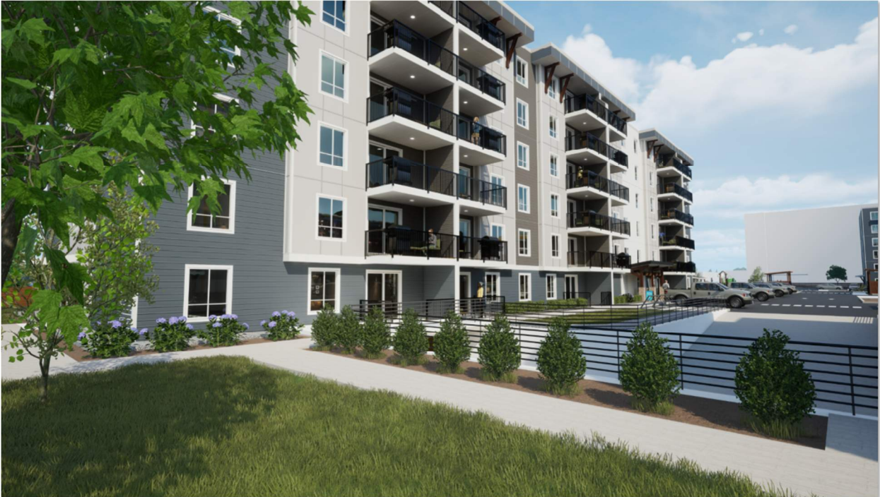
Figure 12: Building D looking northwest
