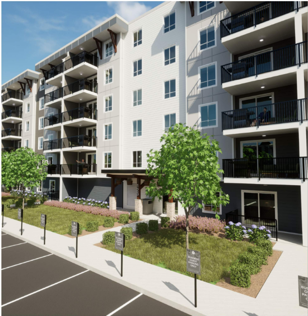
Figure 11: Building B looking north
