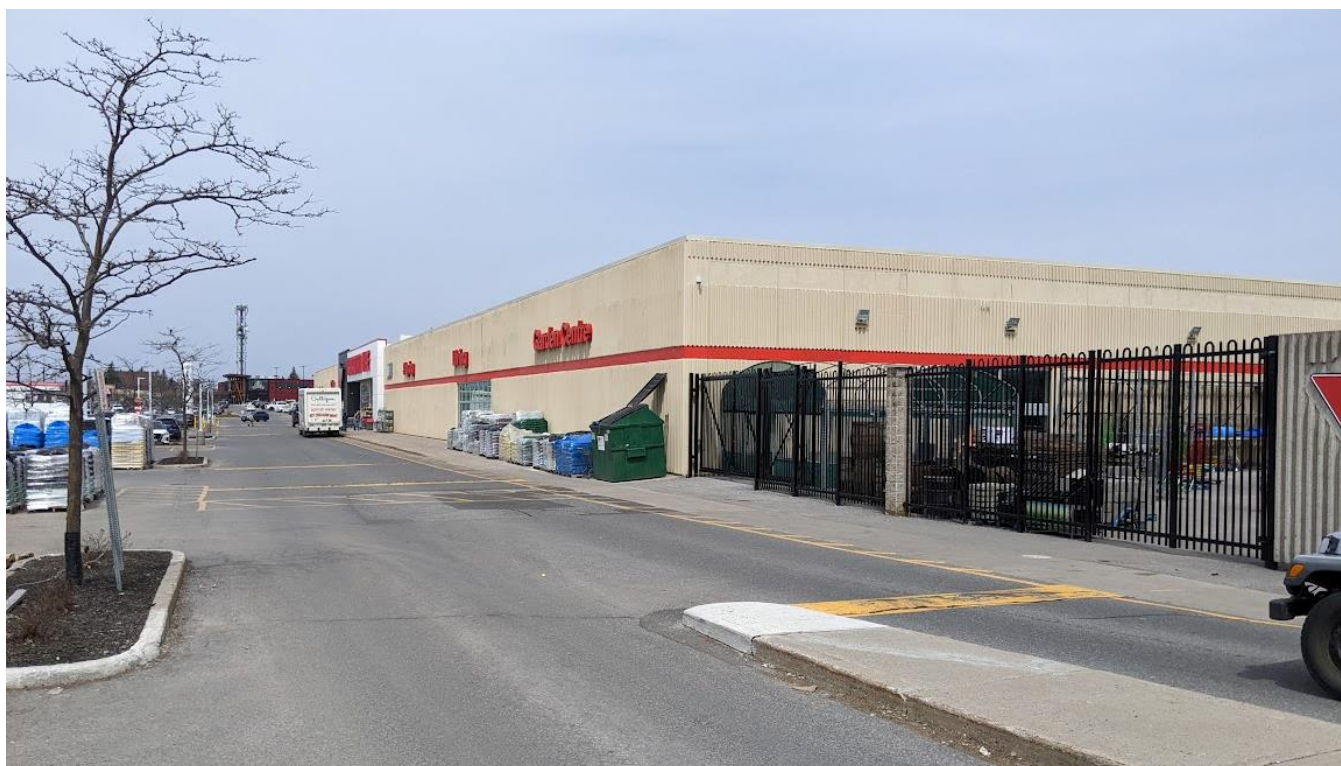
Photo 2: View of existing garden centre and frost house area, looking northeast towards the main building entrance (Parsons, April 2023).
