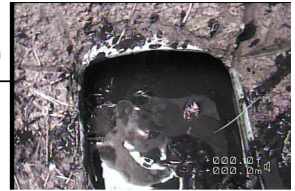
Figure#4: A view to the 40% Debris sediment at 4.6 meters from the top of MHSA1.
