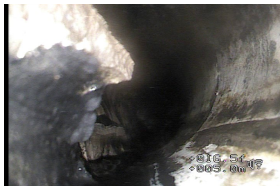
Figure#11: A view to the 5% water level at 6.6 meters from the top of STACKCO (RD1).
