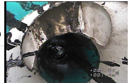
Figure#6: A view to the 40% water level at 2.8 meters from the top of STACKCO (RD1).
