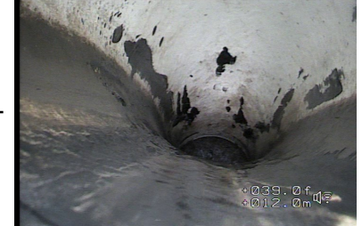
Figure#8: A view to the line deviation downwards at 11.8 meters from the top of MHSA1.
