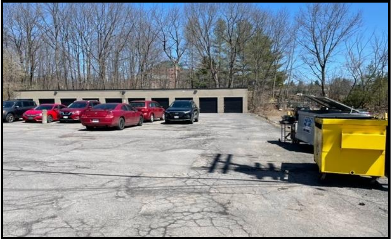
Photograph 3: View of the private parking garage building on the eastern end of the property.
