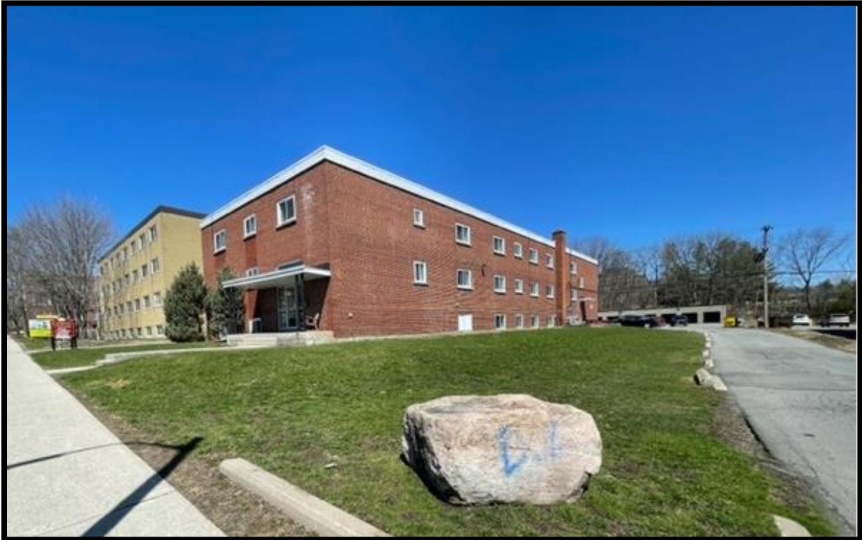
Photograph 1: View of the Phase I Property, taken from Cummings Avenue, looking northeast.
