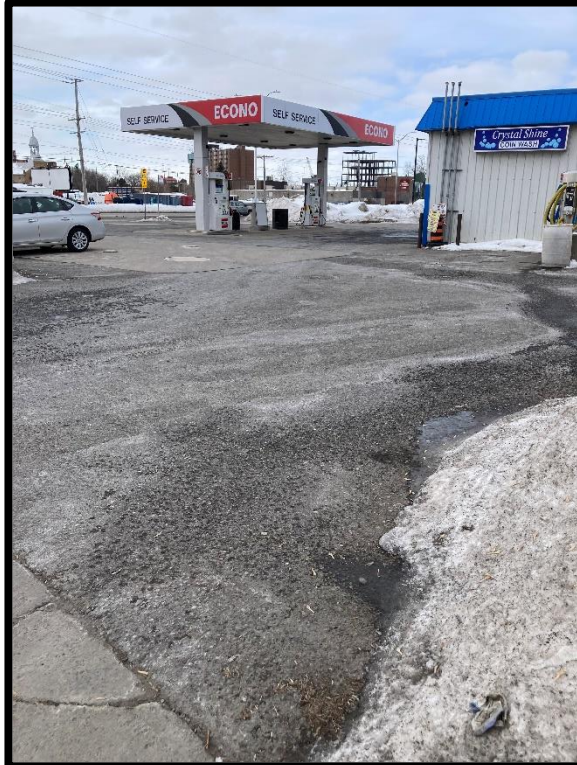
Photograph 8: View of the retail fuel outlet on the 1111 Ogilvie Road property from the southeast corner of the Phase I Property, facing northwest.
