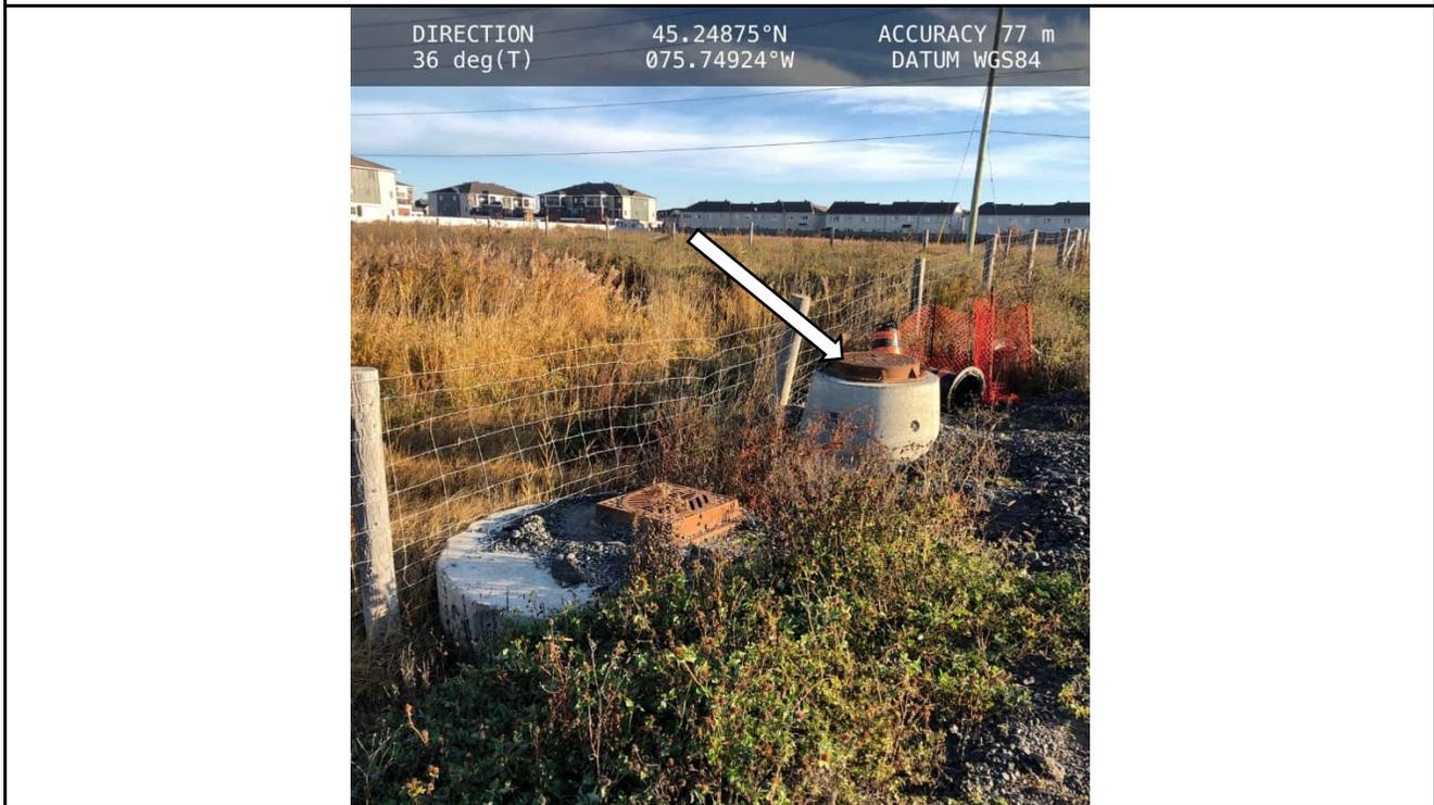
**Photo 6: Storm drain and sanitary manhole (see arrow) observed on-site along southern fence line, facing northeast from the south-central portion of the Site at the Site boundary.**
