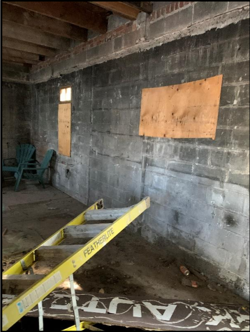
Exposed Masonry Wall Administration Area
