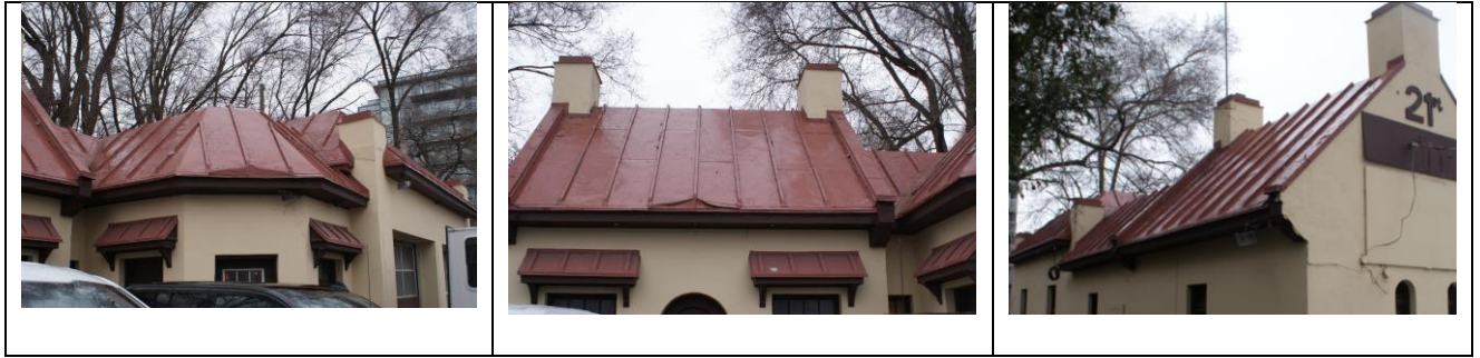
Figure 10: images of the standing seam roofs. Note the diverter flashing treatment above the doors.
