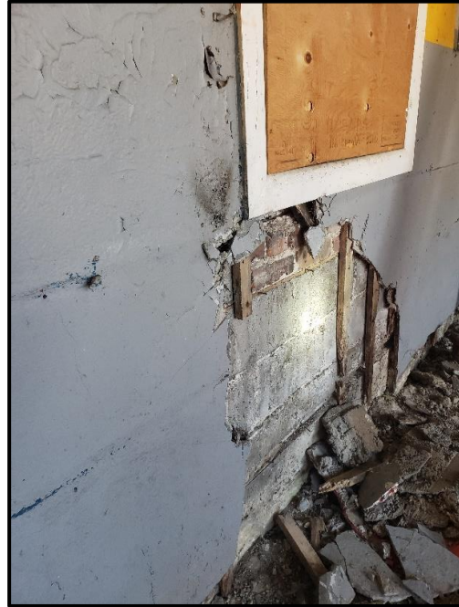
Masonry Wall Behind Plaster Lath - Service Bay
