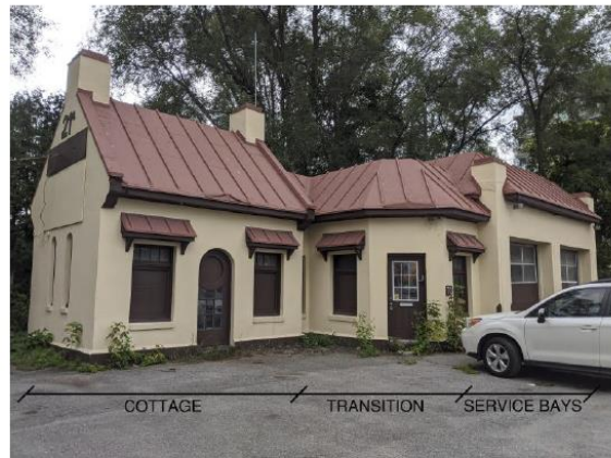
Photo 1: Overview of building [JCAL 2020]
