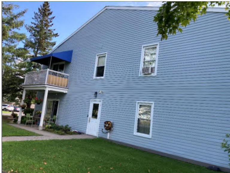
Photo 4 – Site Building (west elevation).
