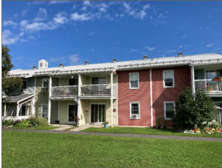
Photo 3 – Site Building (south elevation).
