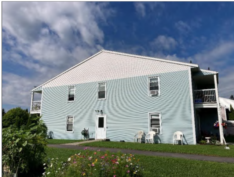
Photo 2 – Site Building (east elevation).
