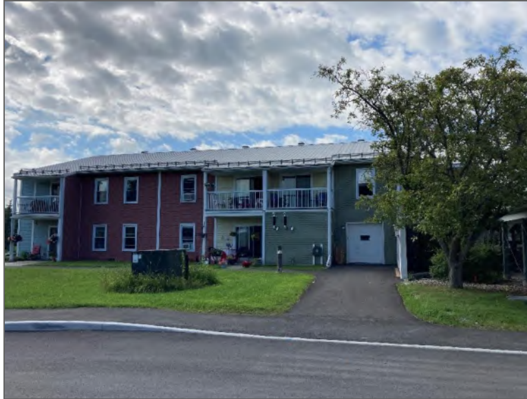
Photo 1 – Site Building (north elevation).
