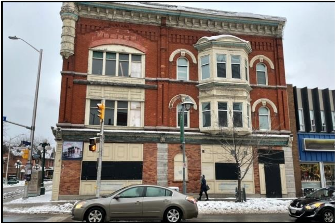
Photograph 1: West view of the Phase I Property, taken from Bank Street.
