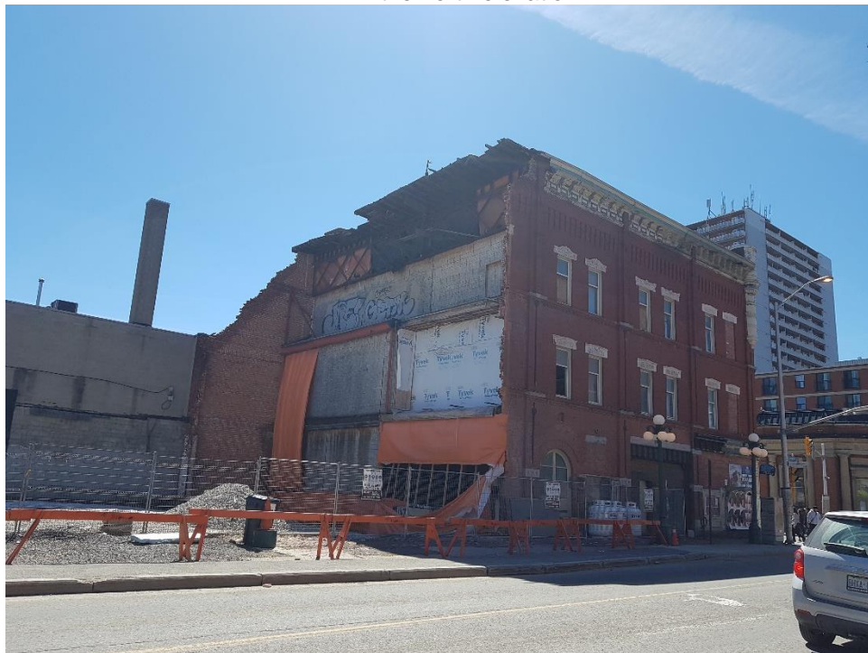
Photograph 6: View of the east elevation. Area is fenced off with restricted access.
