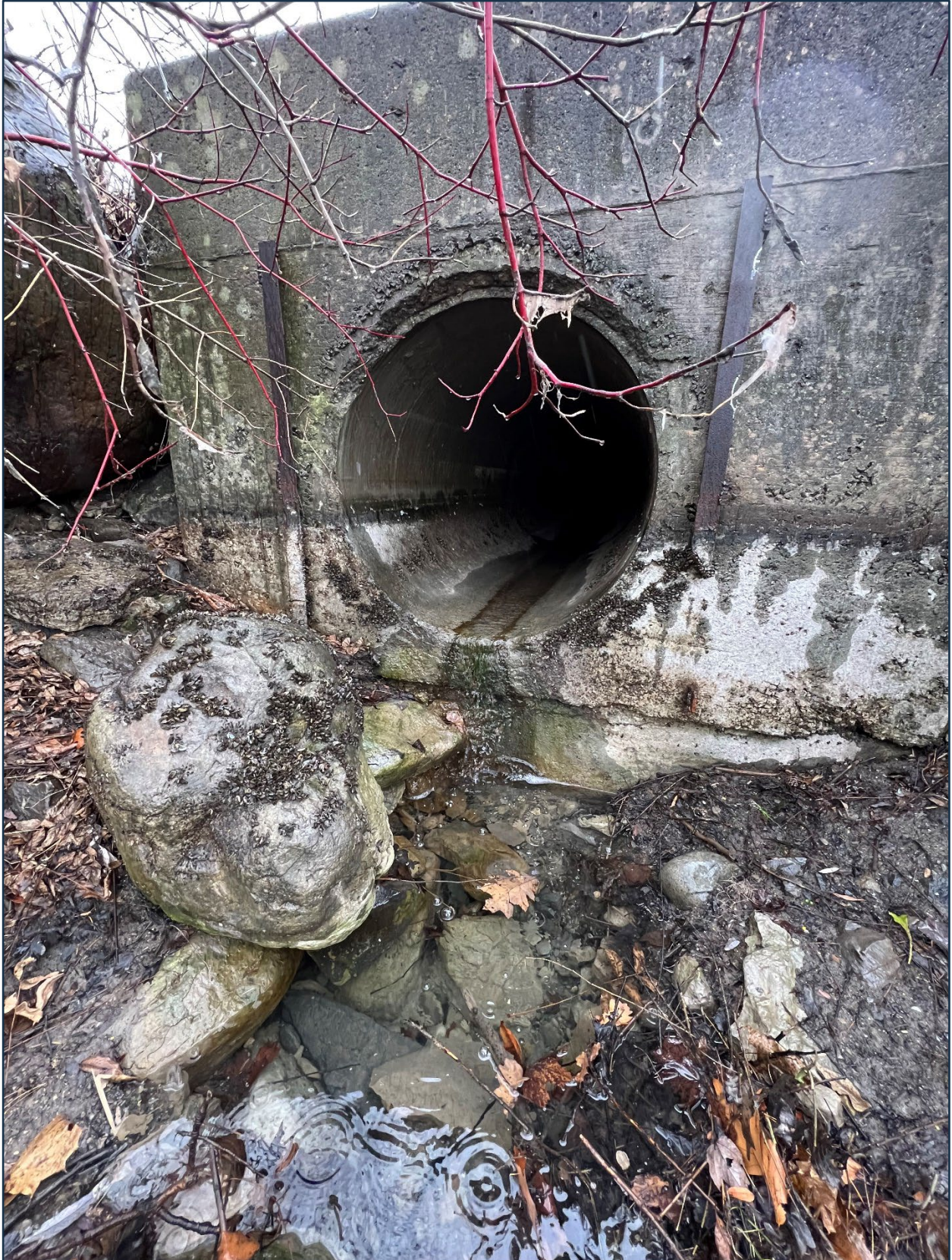
Figure 3-5: Dow's Lake Outfall – December 2022
