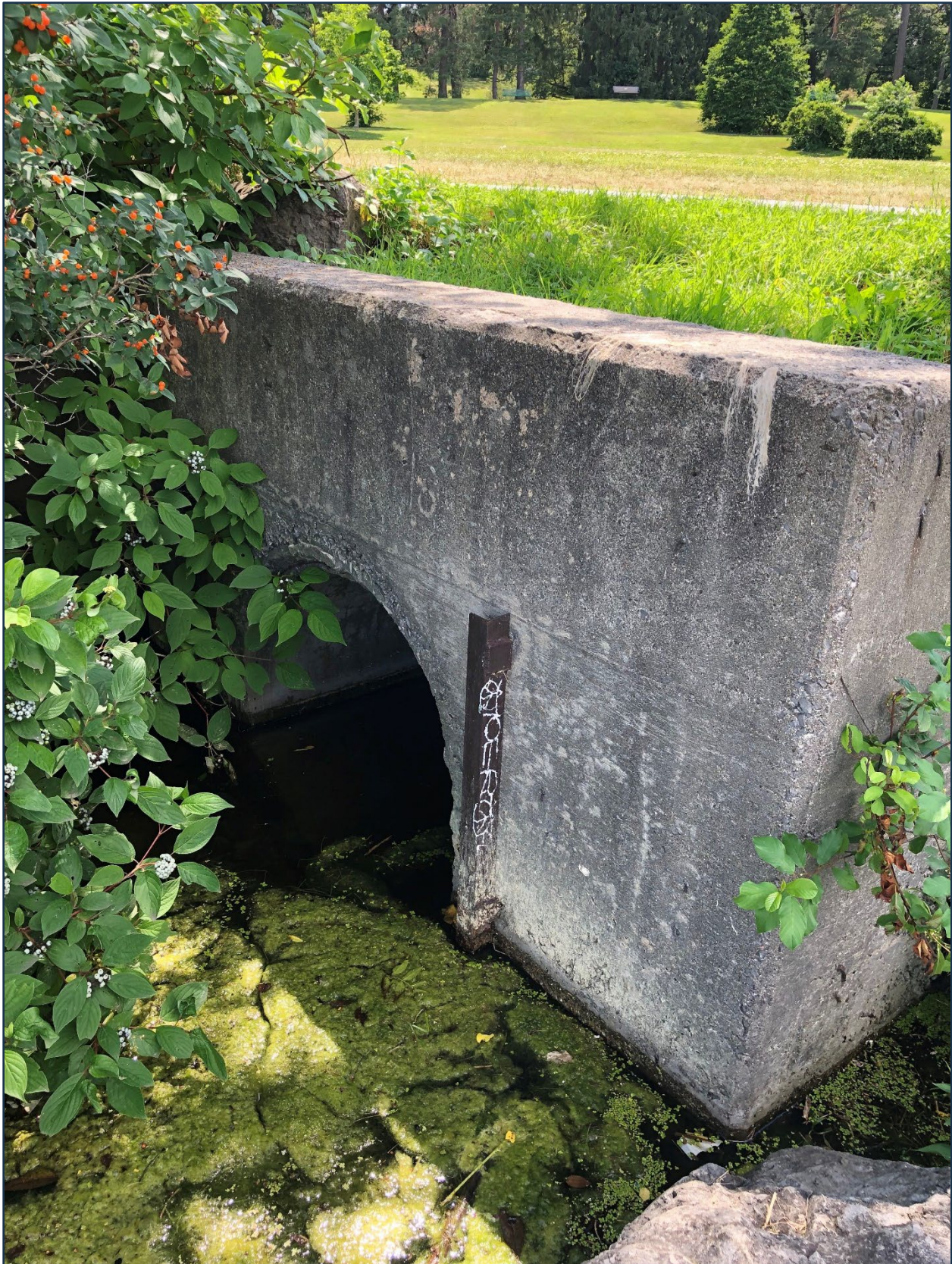
Figure 3-4: Dow's Lake Outfall - July 2022
