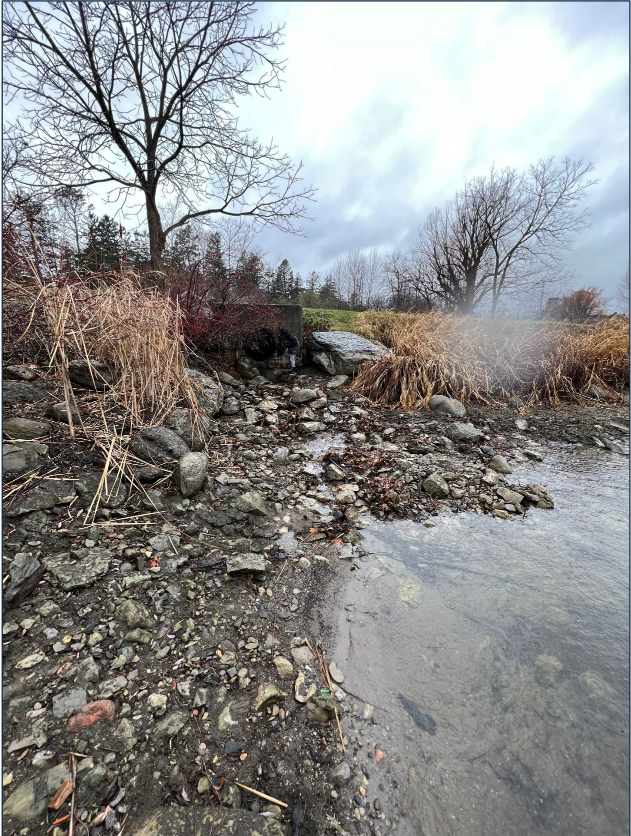
Figure 3-6: Dow's Lake Outfall – December 2022
