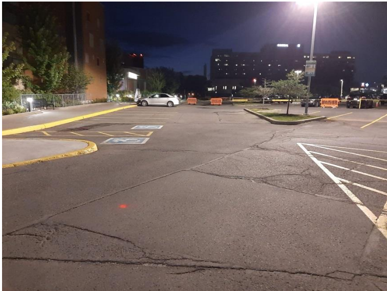
Figure 2 -3: Photo of the north west side of Parking Lot A during survey acquisition.
