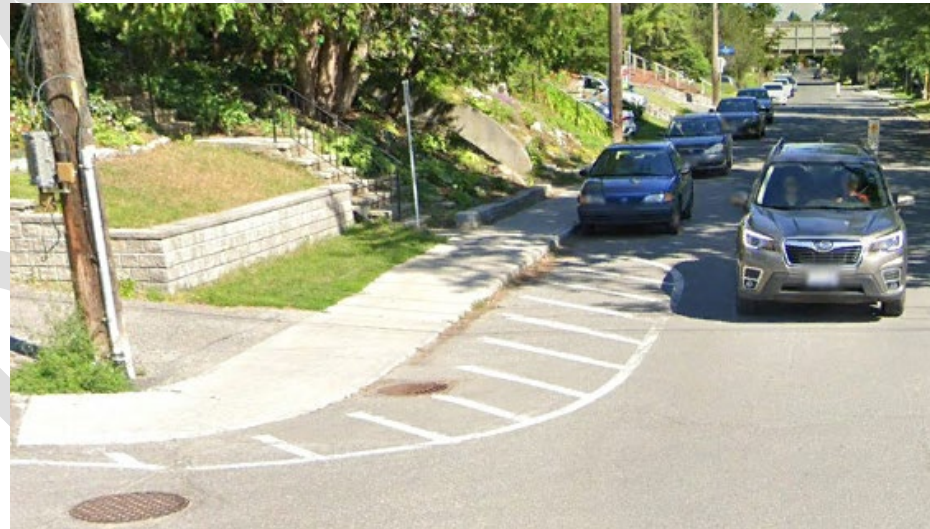
Image: Fairmont Avenue. and Hereford Drive, Ottawa, ON (City of Ottawa, 2022)
