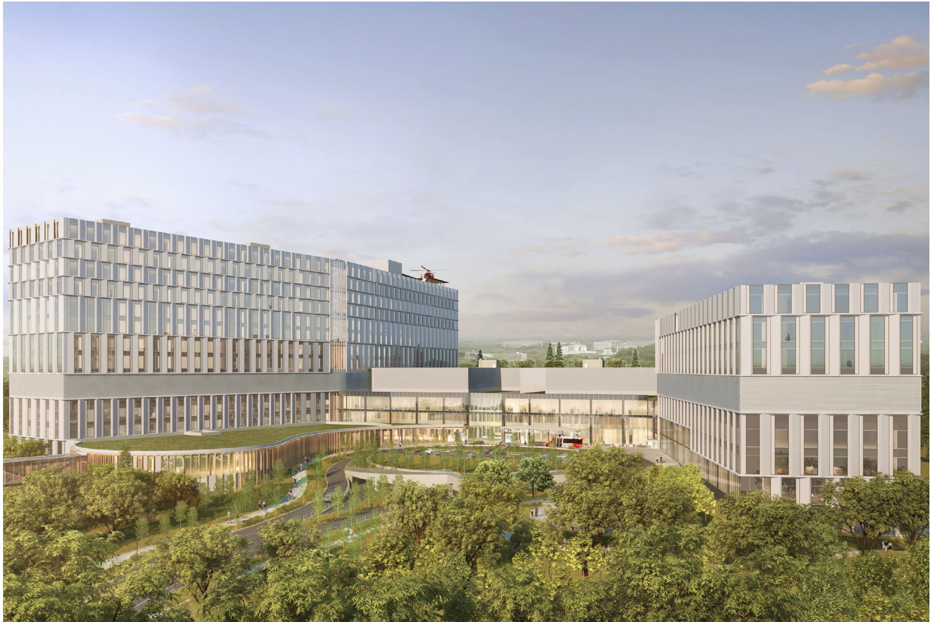
Figure 76: Hospital Main Plaza
