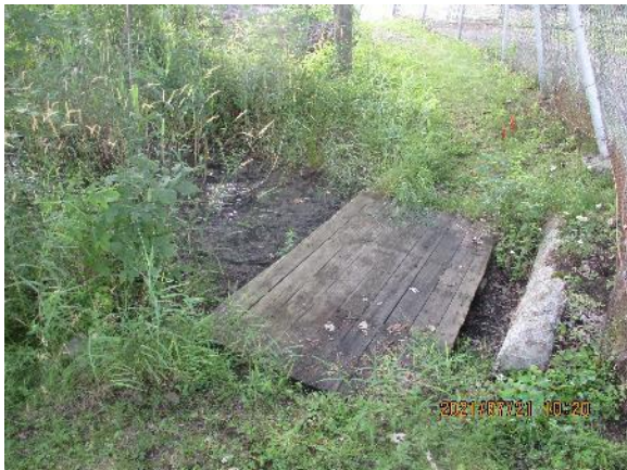
P9 – Wetland area (outlet location, headwall)
