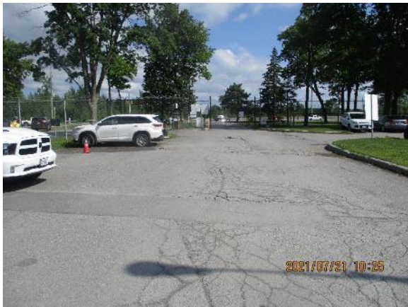
P3 – Fire Route (looking north)
