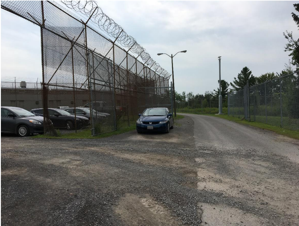
Photograph # 3: View of west side of building, fenced, gravel parking lot space located adjacent to the fire lane
