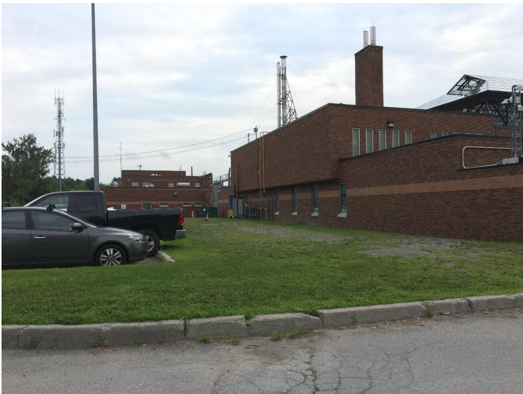
Photograph # 13: View of North side of building at existing parking lot
