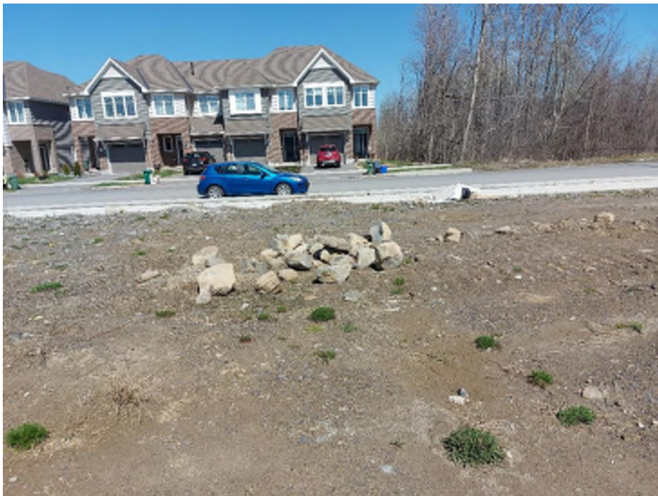
Photograph 2: Onsite fill piles
