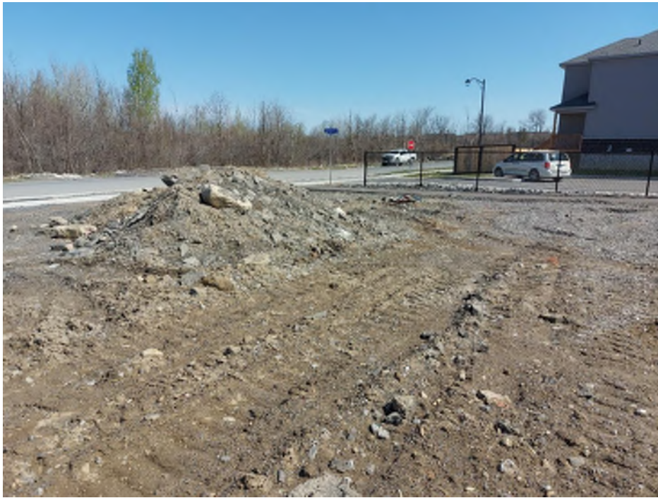
Photograph 3: Additional onsite fill piles
